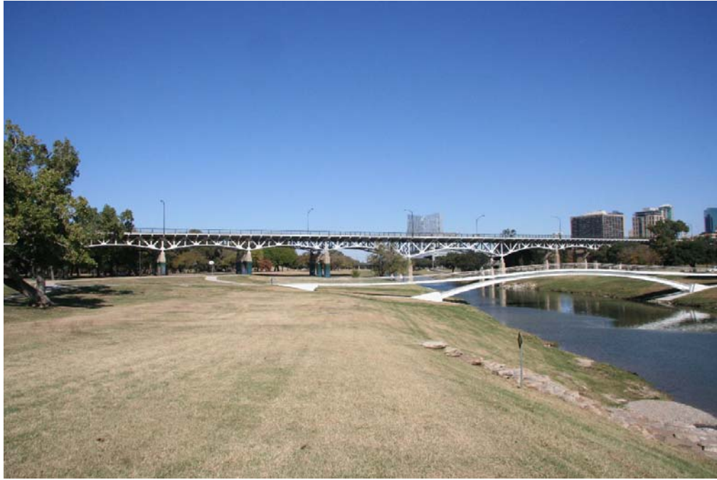
Photo 1: South elevation, facing north, showing the continuous Warren deck truss with variable-depth bottom chord, a rare type
