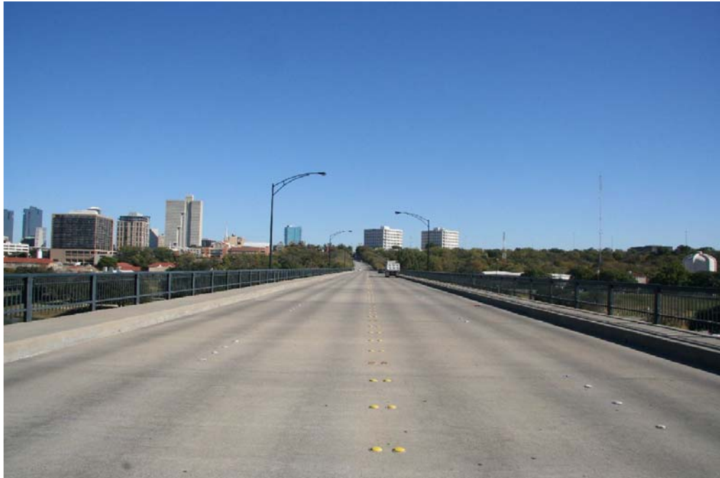
Photo 2: Deck view, facing east
