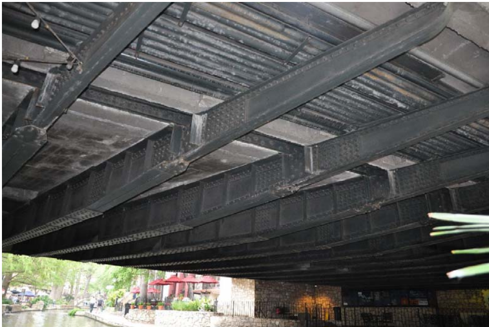
Photo 4: Detail of underside and cantilevered sidewalks; view facing northwest
