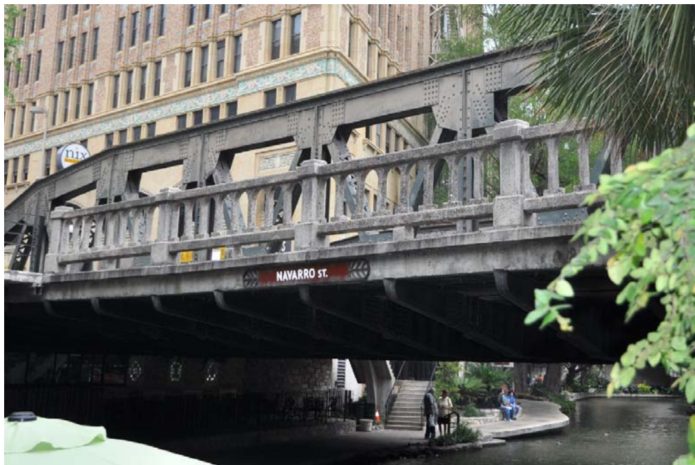
Photo 2: West elevation with original sidewalk railing; view facing northeast
