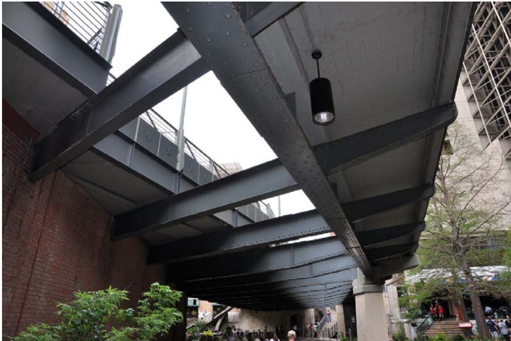
Photo 6: Underside of truss and cantilevered sidewalk, view facing north
