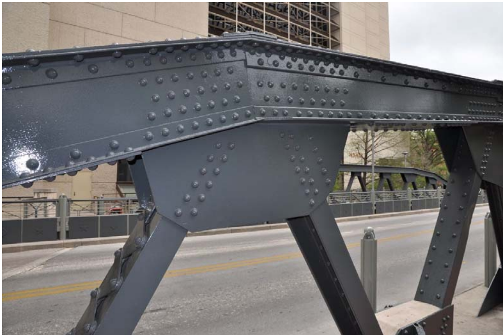
Photo 4: Detail of primary truss connection with rivets, view facing southwest
