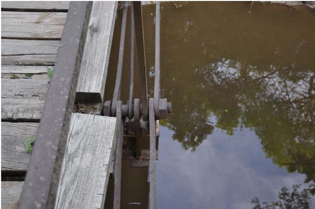
Photo 4: Detail of primary connection at bottom chord and U-bolt at floor beam
