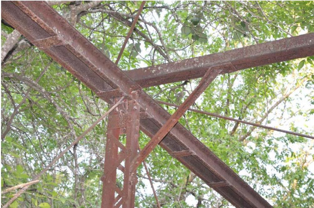
Photo 2: Detail of primary connection at top chord, vertical, and sway bracing
