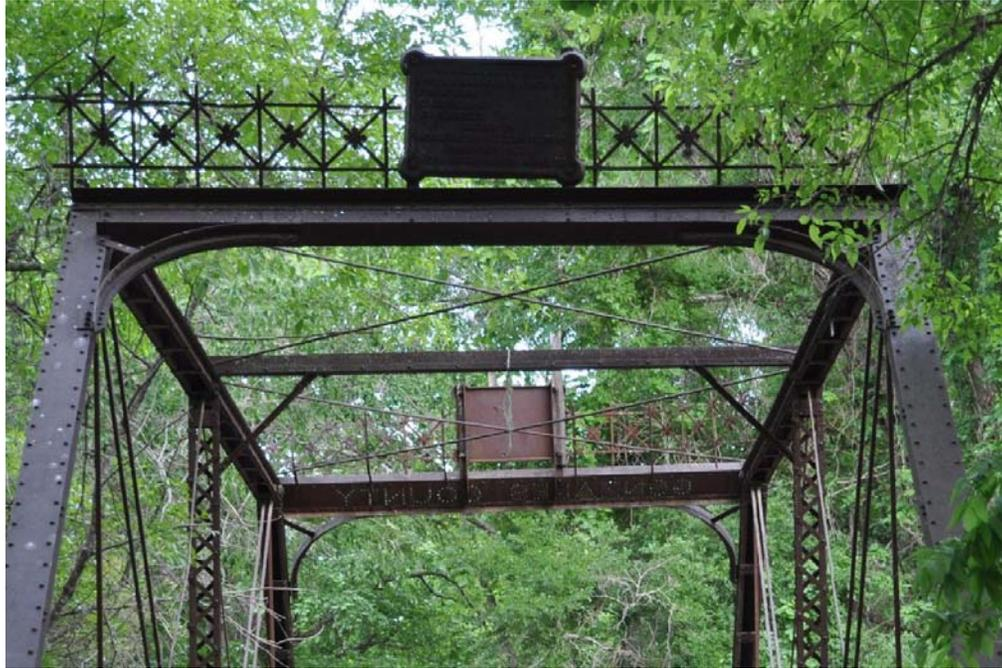
Photo 5: Detail of decorative portal with curved knee bracing, intricate cresting, and punched bracing
