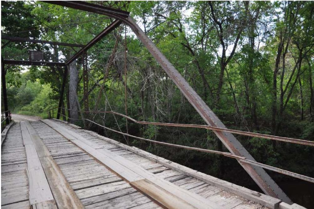
Photo 6: Detail of truss panel with replacement railing
