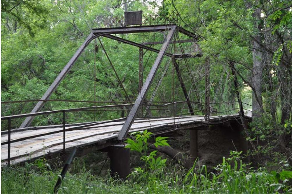
Photo 1: Elevation of one-span, pin-connected Pratt through truss, a rare survivor of a once-common truss type in the state; view facing east-northeast
