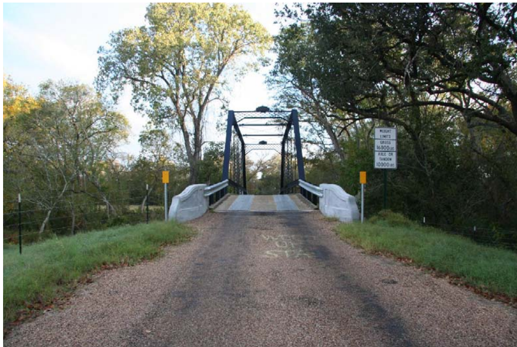
Photo 6: Overview of setting and replace approach span; view facing north
