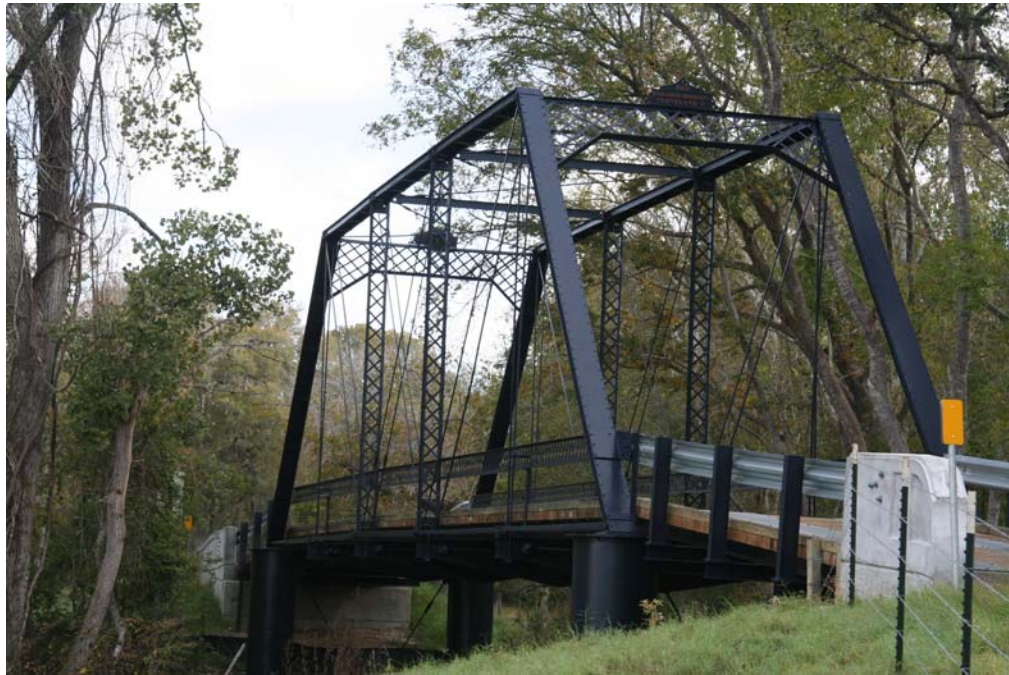
Photo 1: Oblique view of west elevation; view facing northeast
