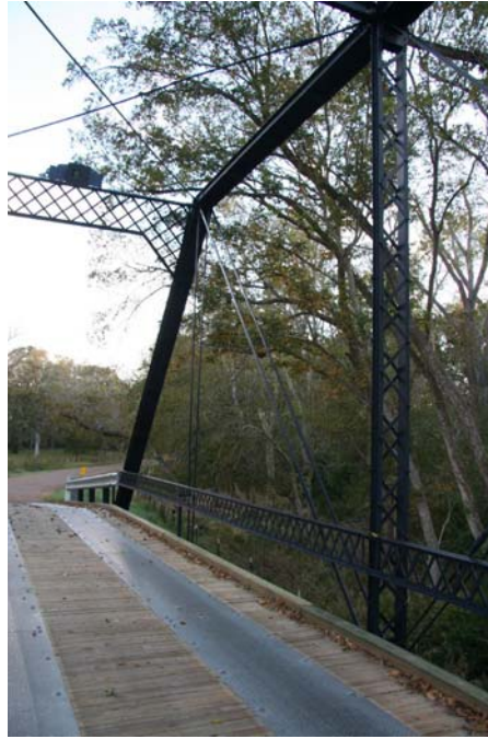
Photo 5: Detail of truss panel and decorative portal; view facing northeast
