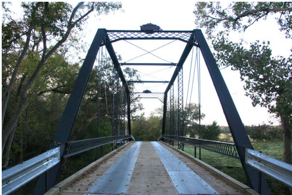
Photo 2: Deck; view facing southwest
