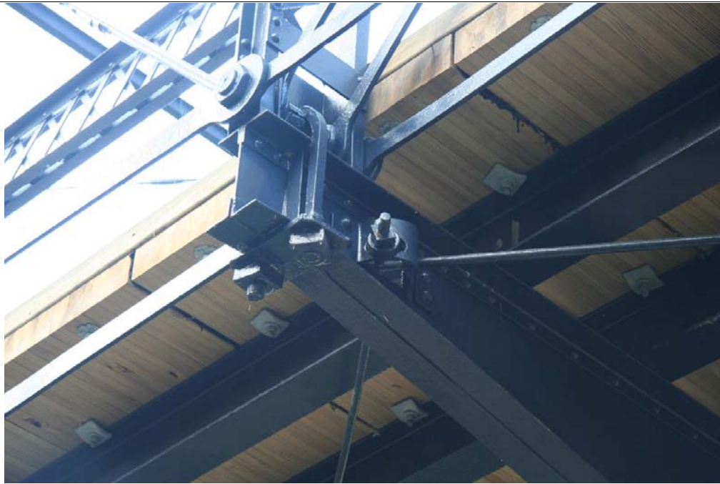
Photo 3: Detail of lower chord pin and floor beam U-bolt connections
