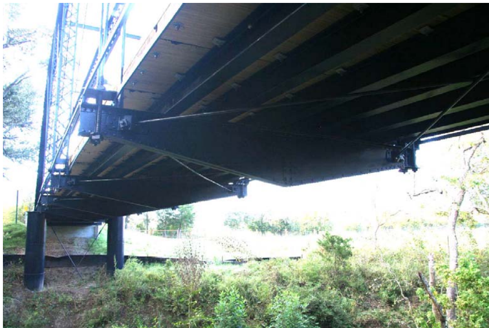
Photo 4: Detail of floor system and fish-belly beams; view facing southwest
