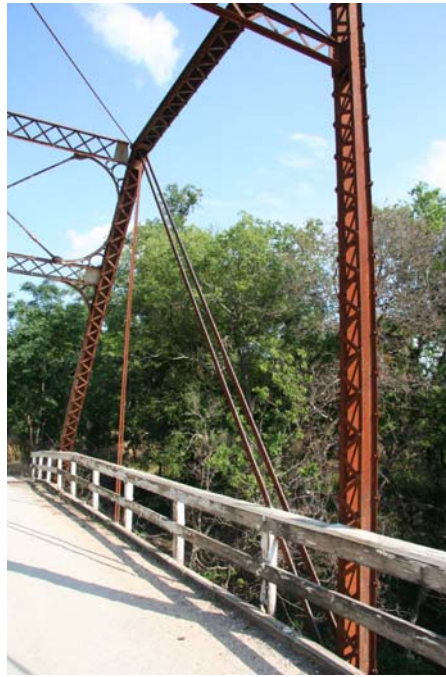
Photo 5: Detail of truss panel; view facing northwest
