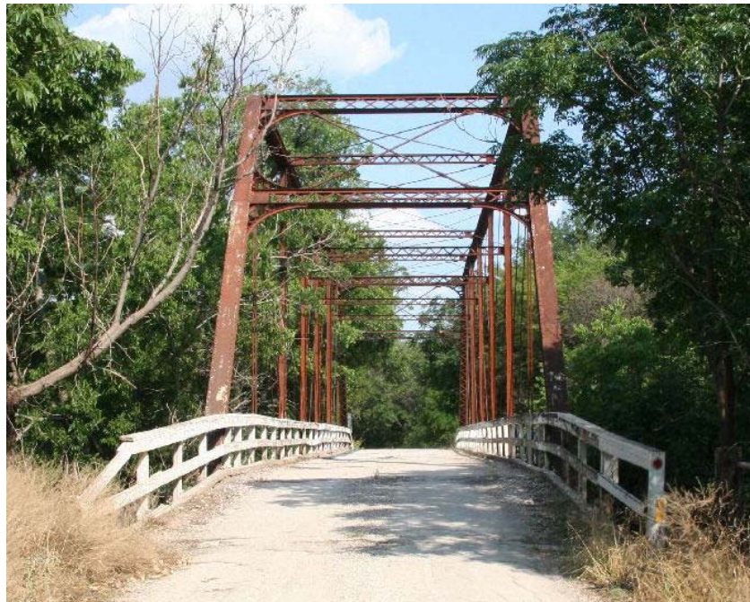
Photo 4: Overview of deck and approach roadway; view facing east
