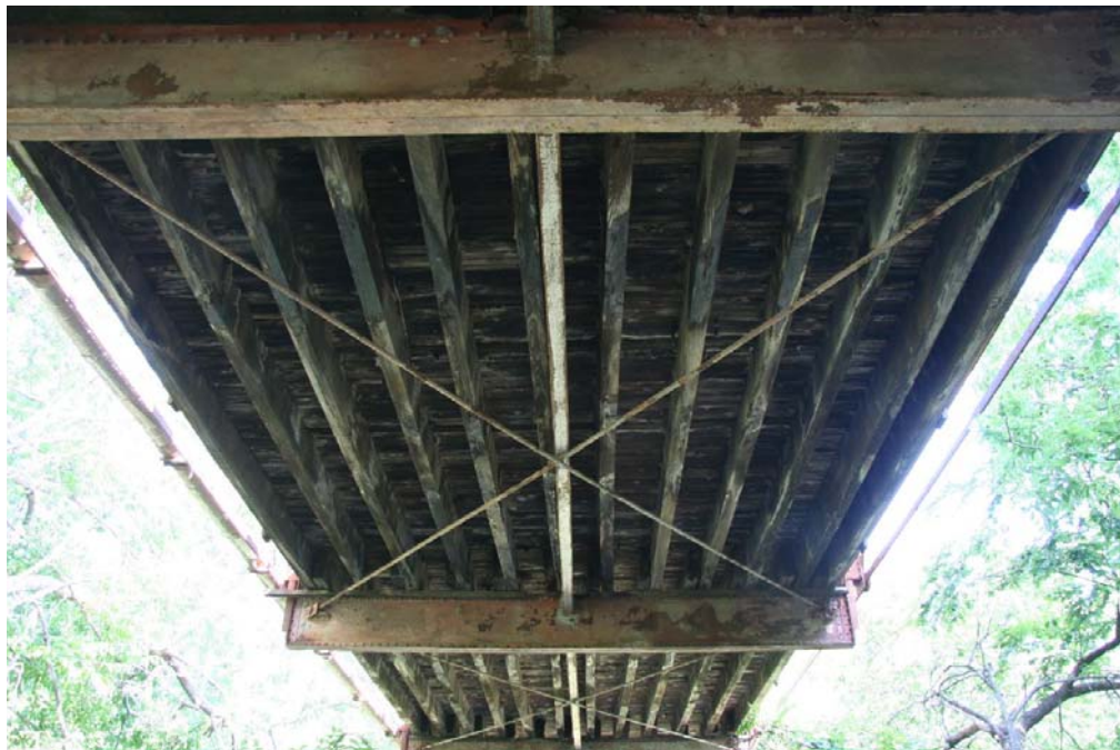
Photo 6: Underside of truss; view facing east
