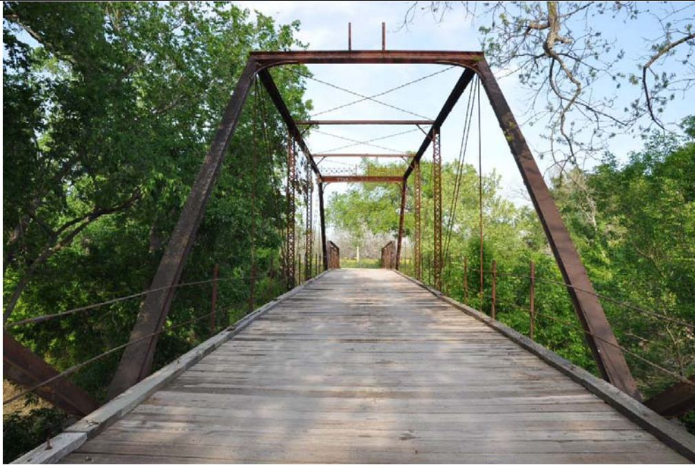
Photo 3: Overview of truss panel on main span; view facing northeast
