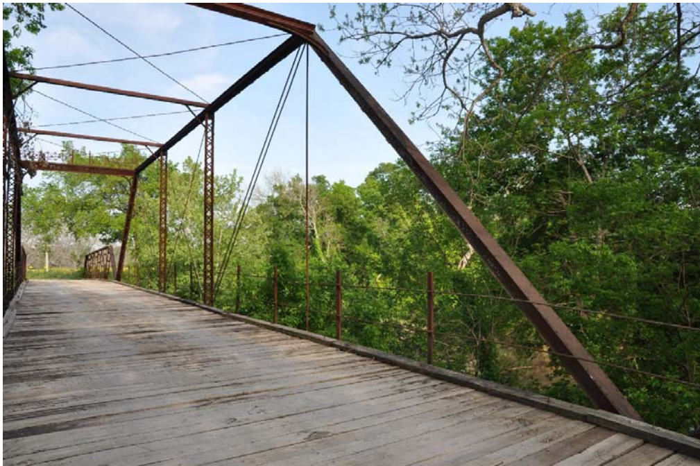
Photo 4: View of main pin-connected Pratt through truss span; view facing east
