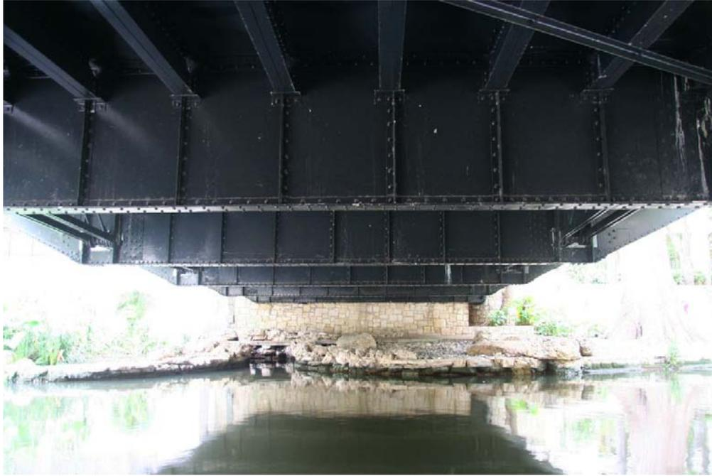
Photo 5: View of underside of truss, facing east, showing built-up floor beams, stringers, and bottom chord with pin connections
