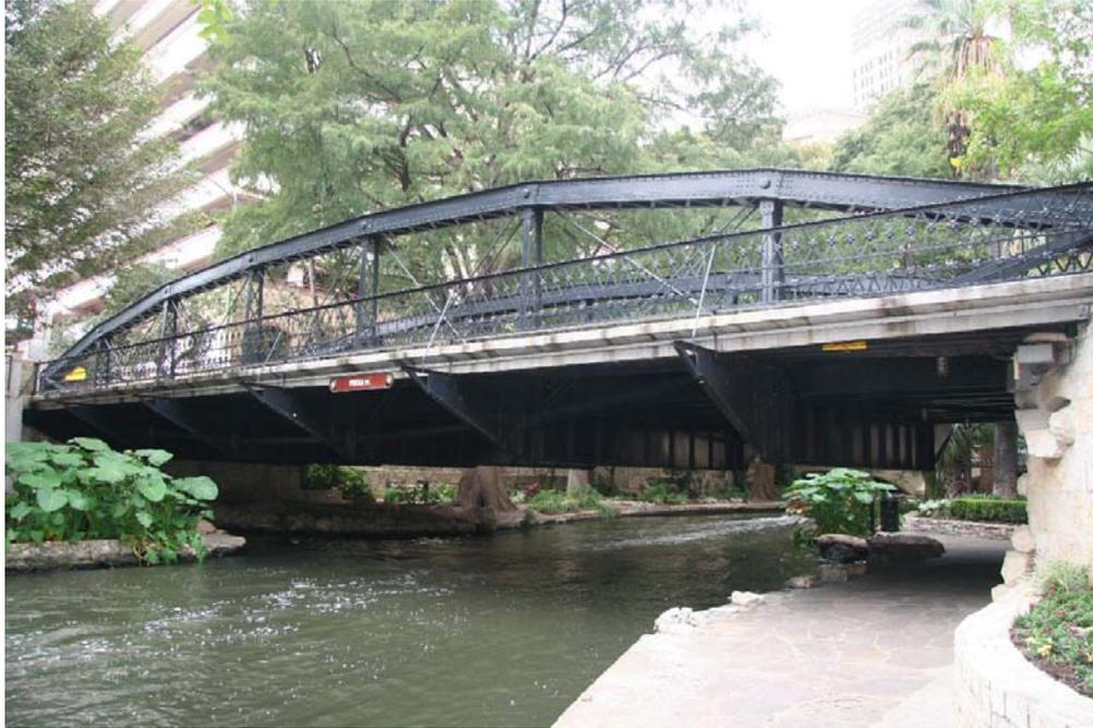
Photo 1: North elevation, facing south, showing the lenticular design of the top and bottom chords that comprise the significant truss type; this is one of the few known examples in the state
