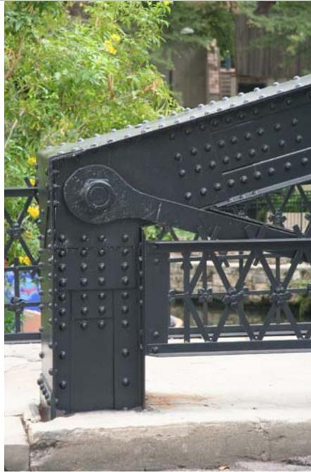
Photo 3: Detail of pin connection joining top chord, bottom chord, and lenticular end post
