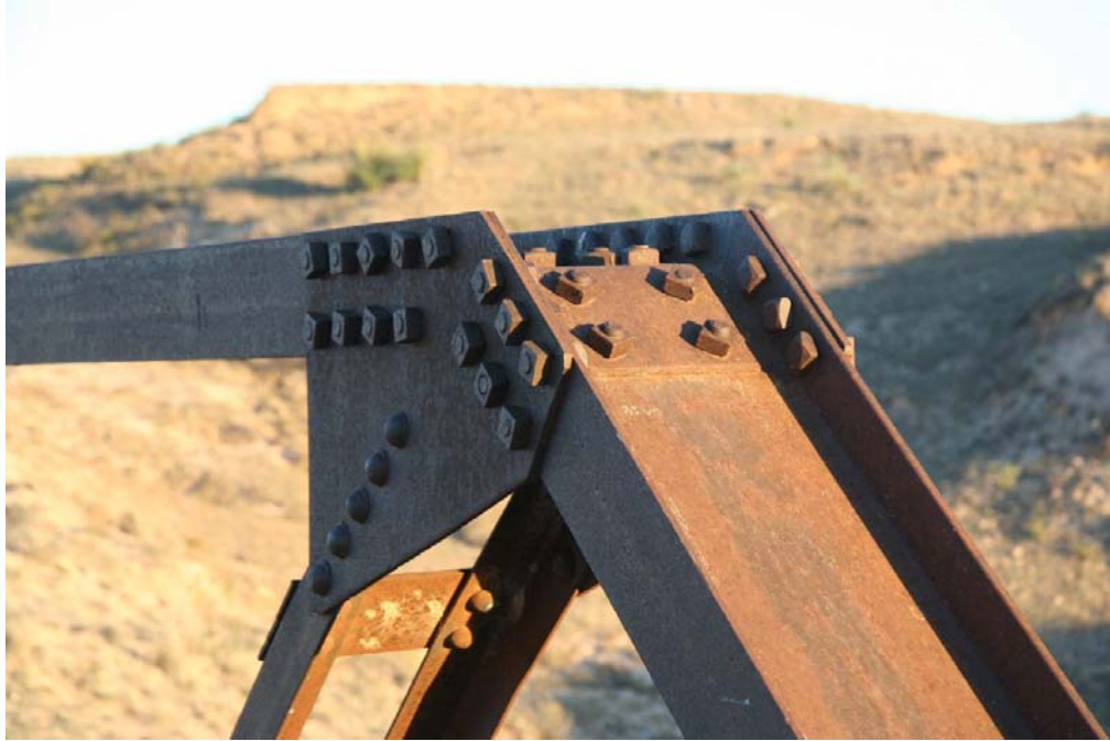
Photo 3: Detail view of top chord connection
