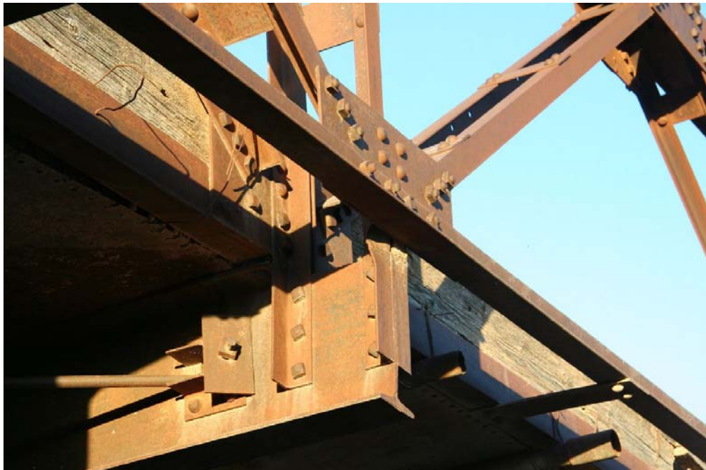
Photo 4: Detail view of bottom chord connection with floor beam
