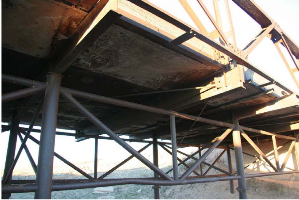
Photo 5: Oblique view of supplemental substructure, facing northeast
