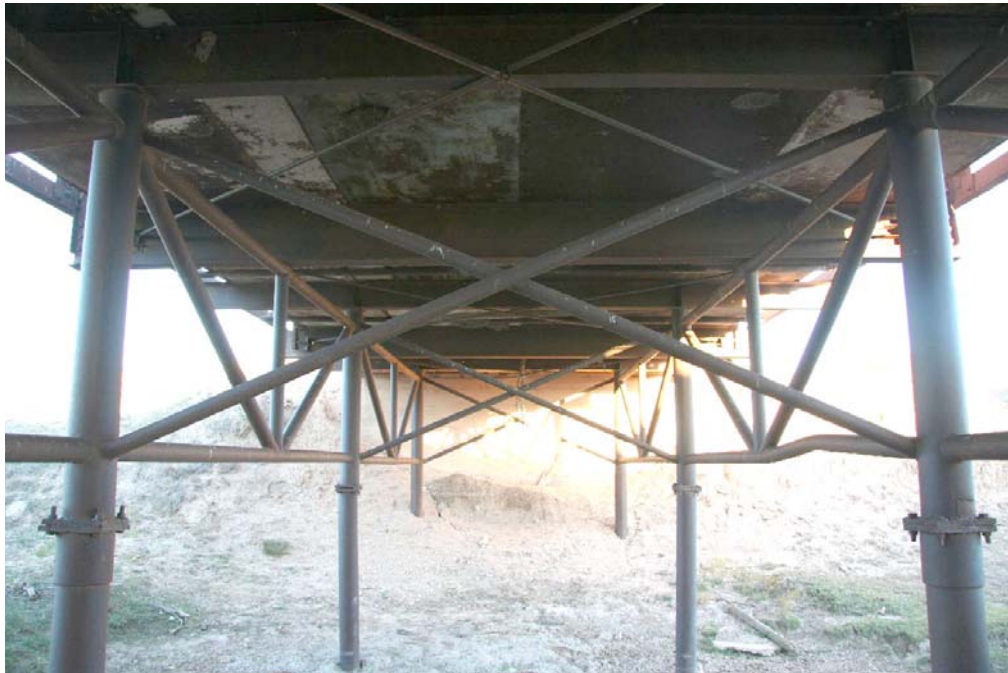
Photo 6: View of truss underside, showing supplemental substructure, facing east
