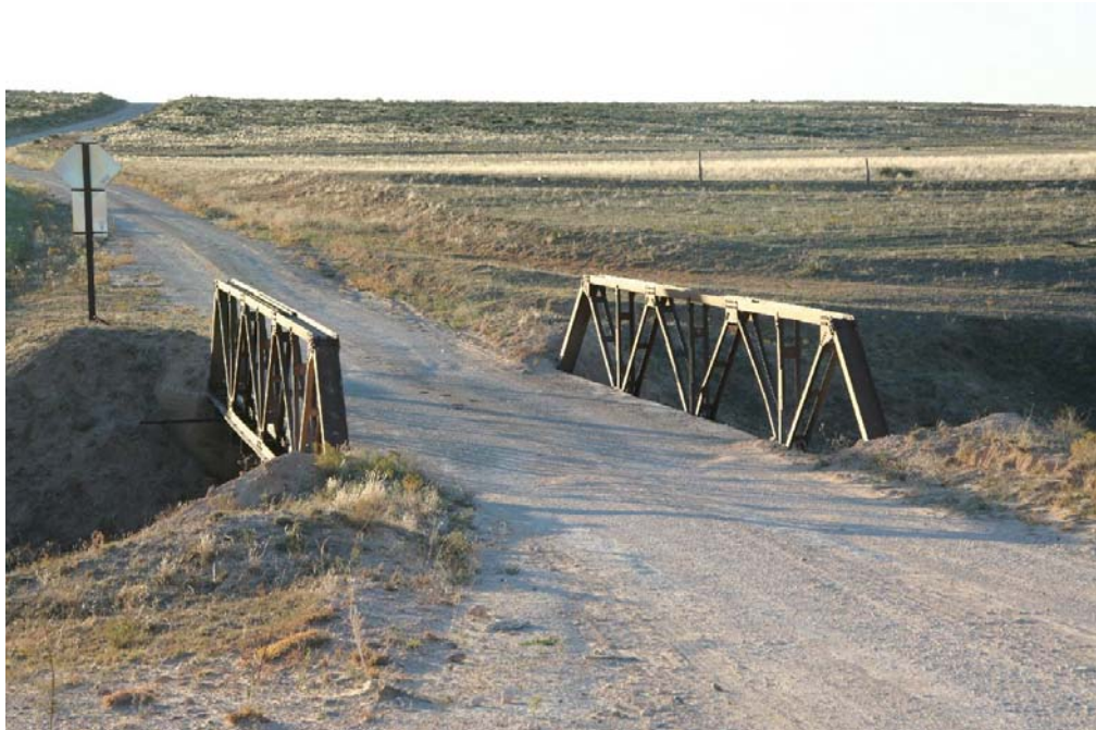
Photo 2: Oblique deck view, facing west
