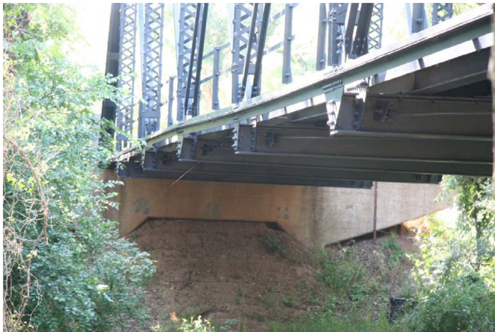
Photo 4: Detail of bottom chord and primary structural connections
