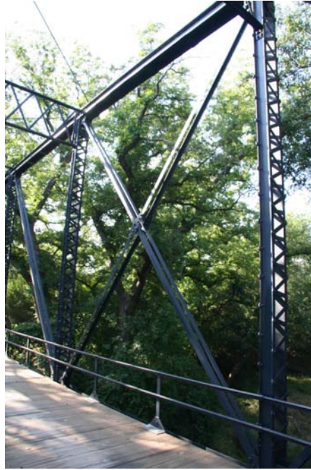
Photo 5: Detail of truss panel
