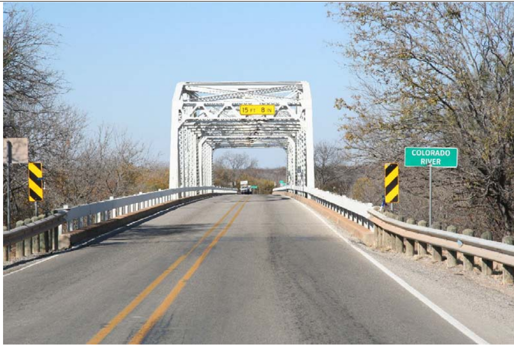
Photo 3: Overview of deck and approach; view facing north
