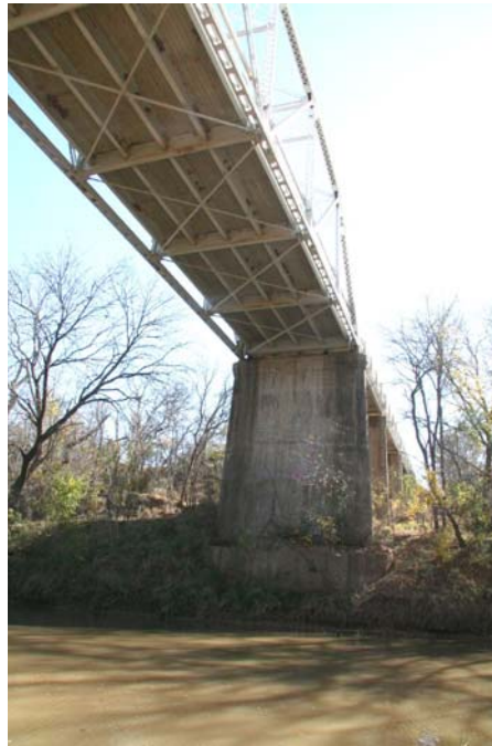
Photo 6: Underside of north truss span and south pier; view facing south
