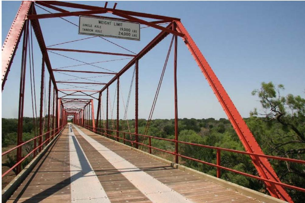
Photo 2: View of pin-connected Pratt through truss spans, view facing southwest
