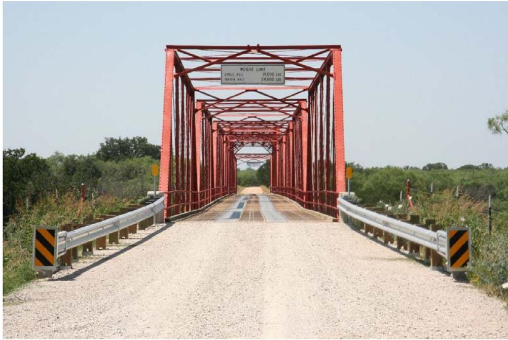
Photo 1: Deck view of the six-span, pin-connected Pratt through truss bridge, a rare survivor of a once common truss type; view facing south
