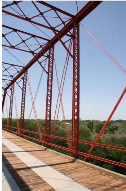
Photo 5: Detail of main span panels where two panels were combined into one to shorten span length
