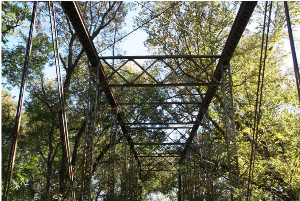
Photo 5: Overview of sway and lateral bracing; view facing east
