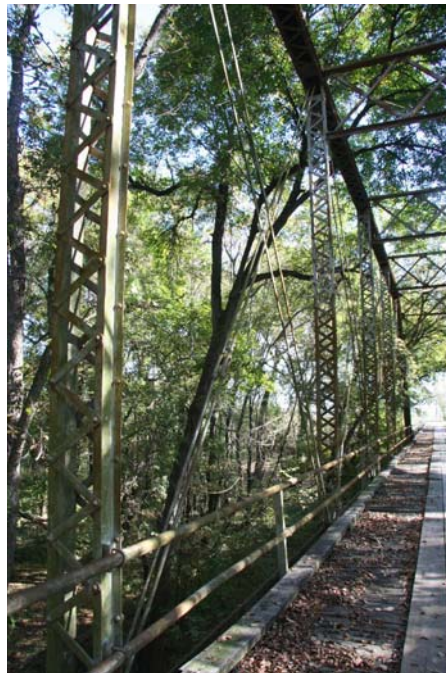
Photo 2: Detail of south truss, showing Pratt through truss configuration and truss members; view facing northeast
