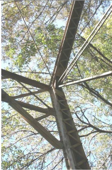
Photo 3: Detail of primary connection at top chord, end post, and portal bracing
