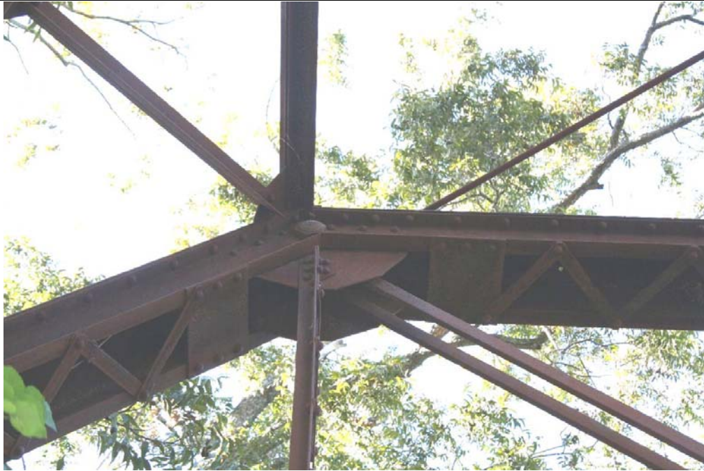
Photo 3: Detail of primary connection at top chord and end post
