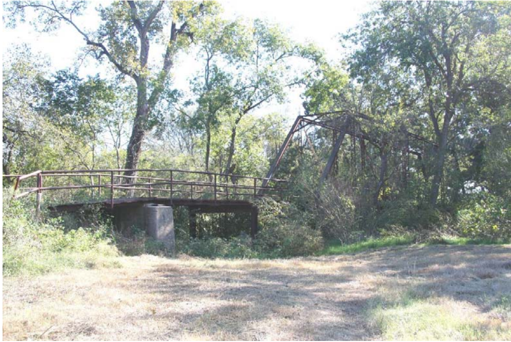
Photo 1: Elevation of one-span, pin-connected Pratt through truss, a rare survivor of a once-common truss type; view facing southeast
