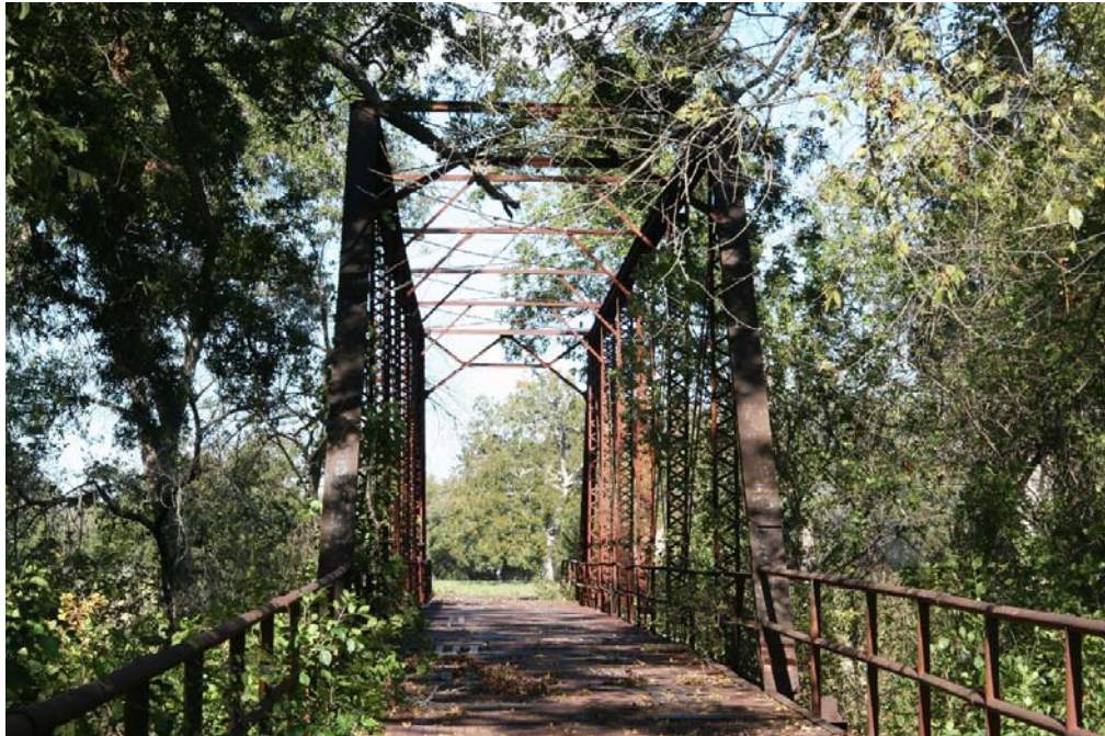
Photo 2: Overview of truss and approach roadway; view facing north
