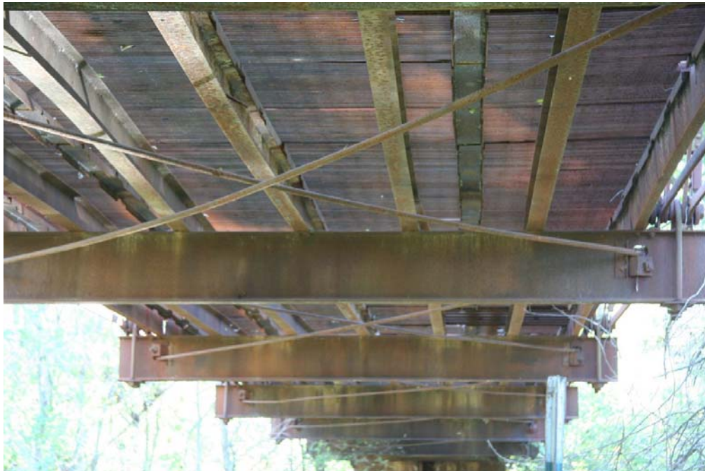
Photo 6: Underside of truss; view facing south
