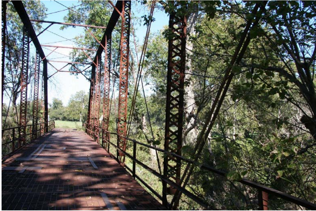
Photo 5: Overview of truss panels, including replacement railing
