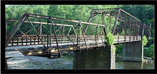
Arroyo Road Bridge: Three spans with variety.
