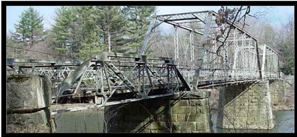
Shanley Road Bridge: Four spans of beauty in metal and stone.
