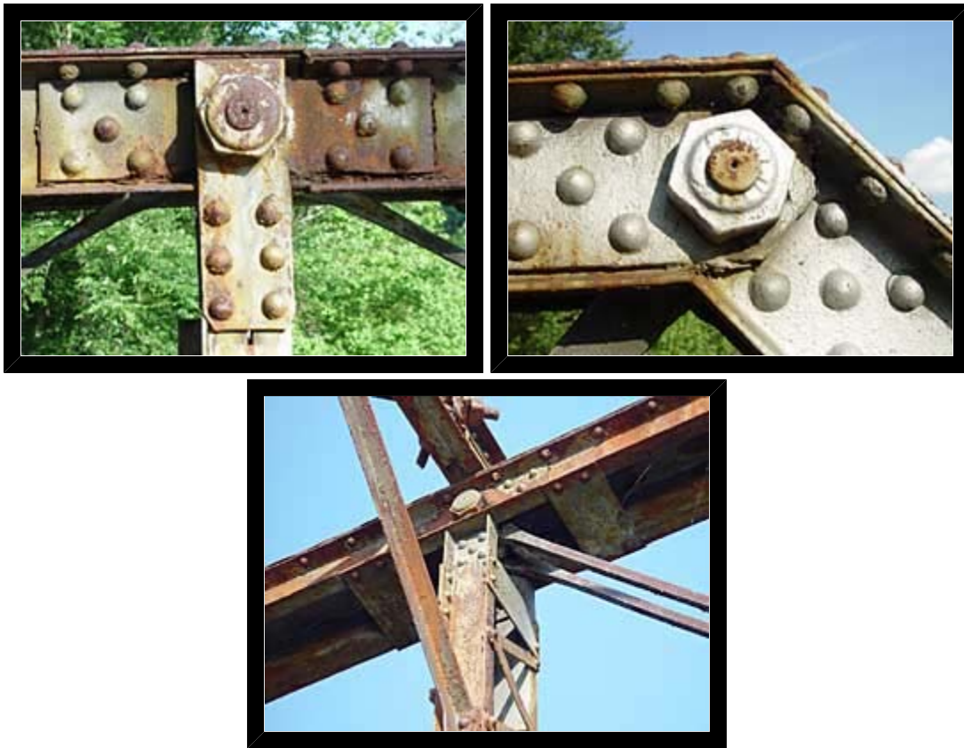
Looking at the Arroyo Road Bridge up close
