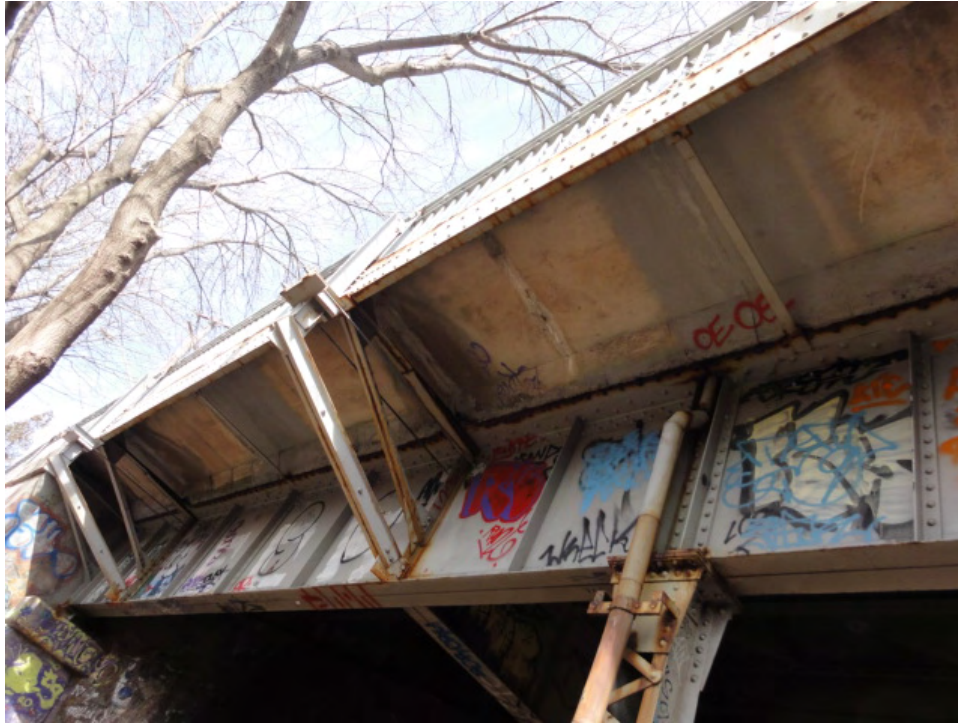
Plate 21: View of steel girders and bracket supports under sidewalks.
