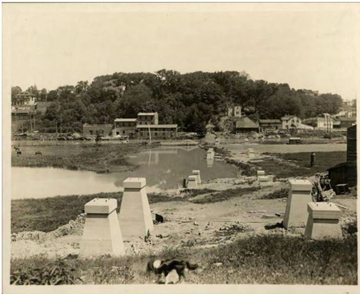
Figure 8: View of the bridge crossing with the concrete piers in place, looking north.
