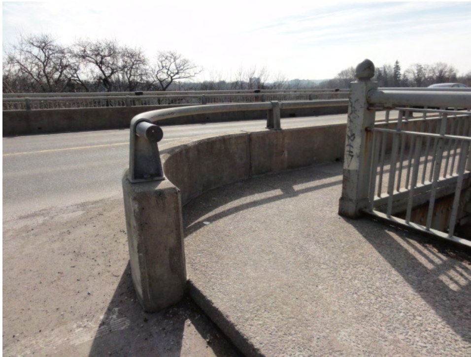
Plate 30: Curved concrete barrier wall with steel hand railing, north approach. Note the open steel hand rails and decorative newel post.
