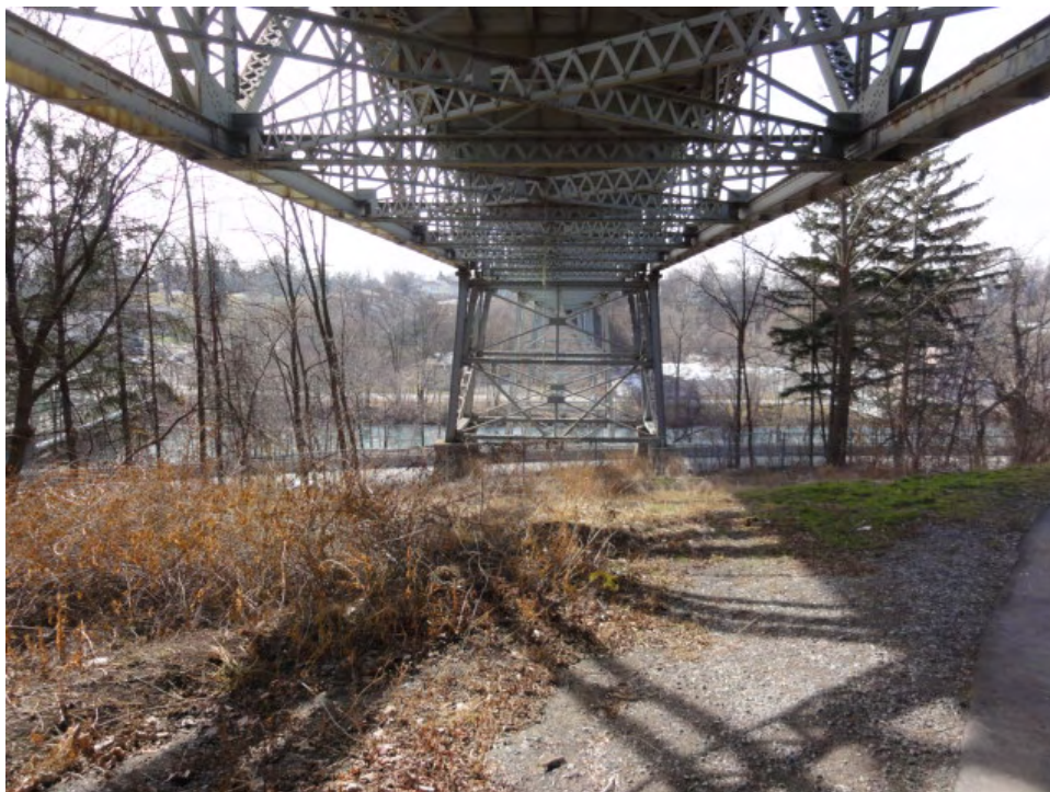
Plate 18: View of deck truss and steel bents resting on concrete pedestals.
