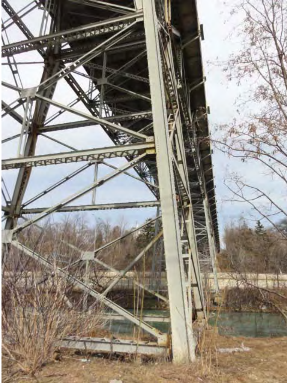
Plate 24: Detail of steel bent support system, south side of Twelve Mile Creek, looking north.
