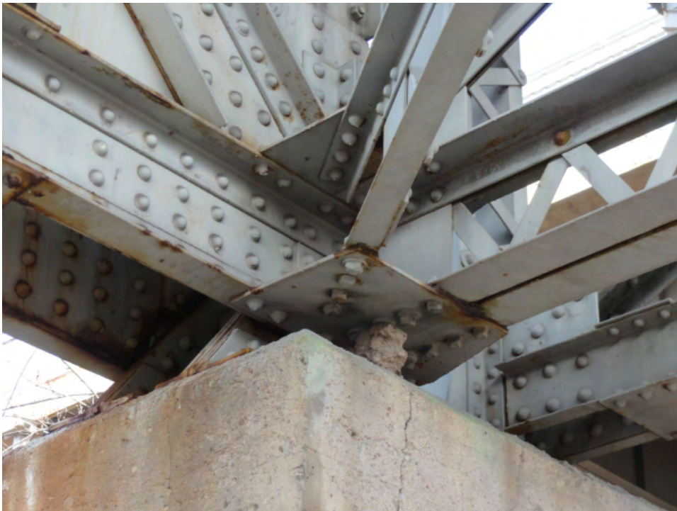
Plate 27: Detail of steel members and mixture of bolted and riveted connections.
