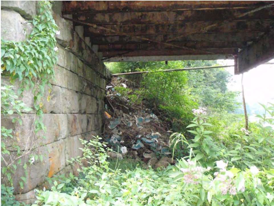
Materials deposited under Carlton Truss.
