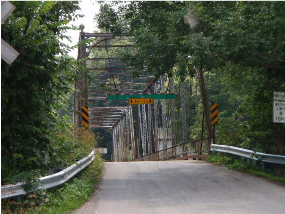
North side of Carlton Truss facing south.
