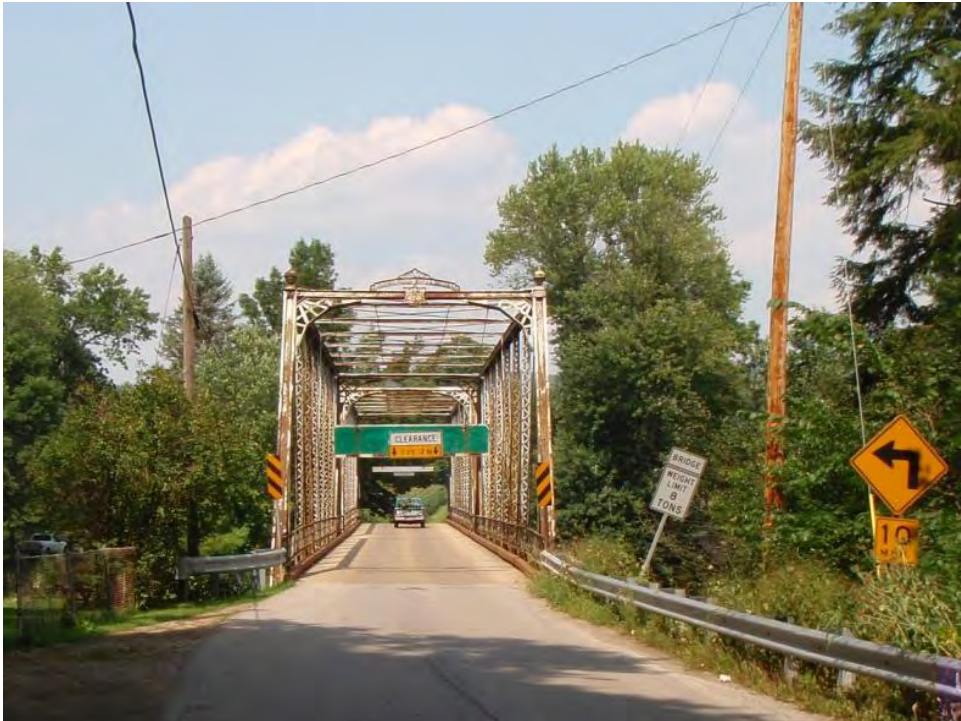
South side of Carlton Truss facing north.
