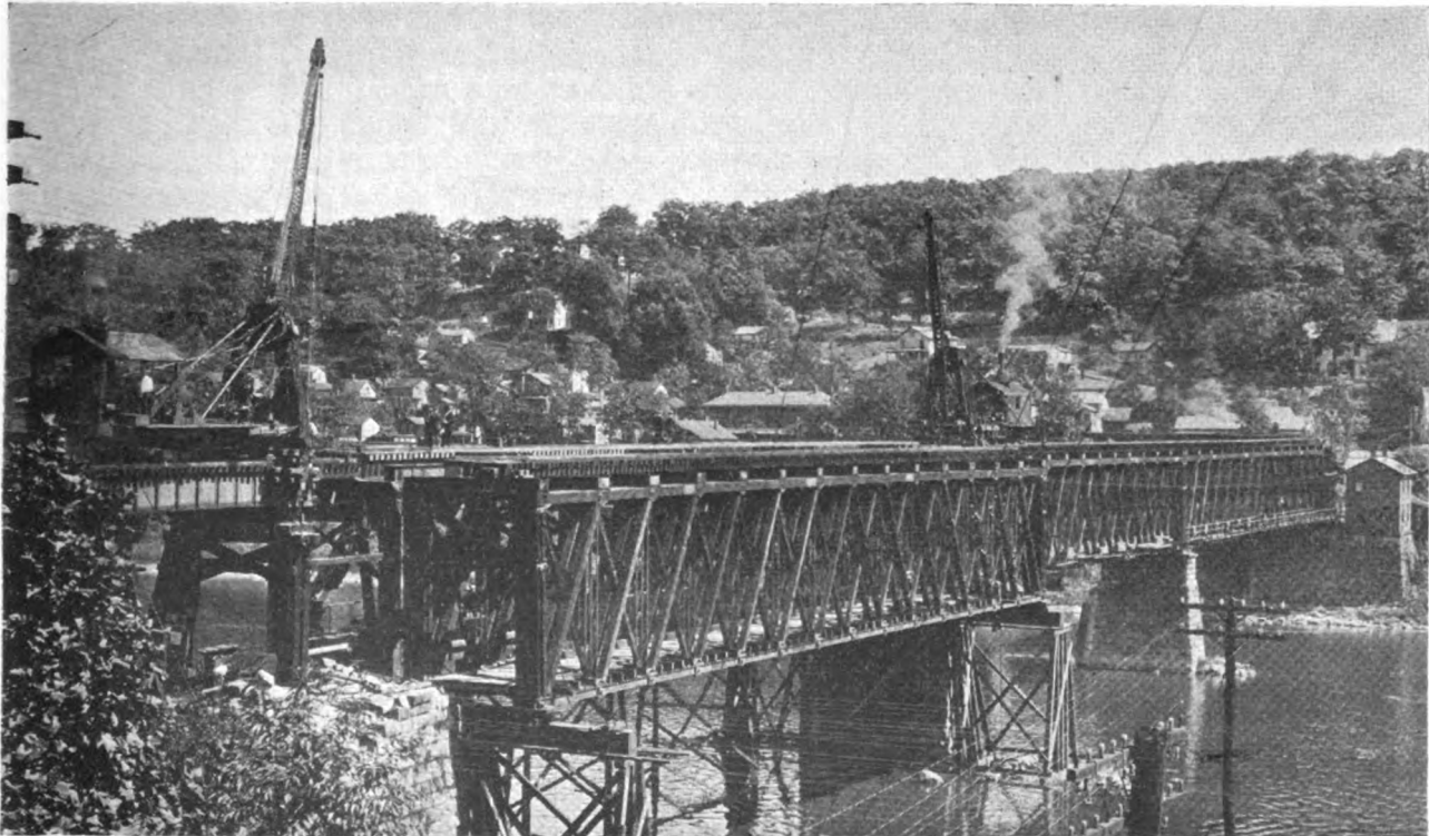
Foxburg Bridge—General view of structure from east end, after conclusion of rolling operation, August 21, showing old span in rolled-out position on falsework, and new span in place
