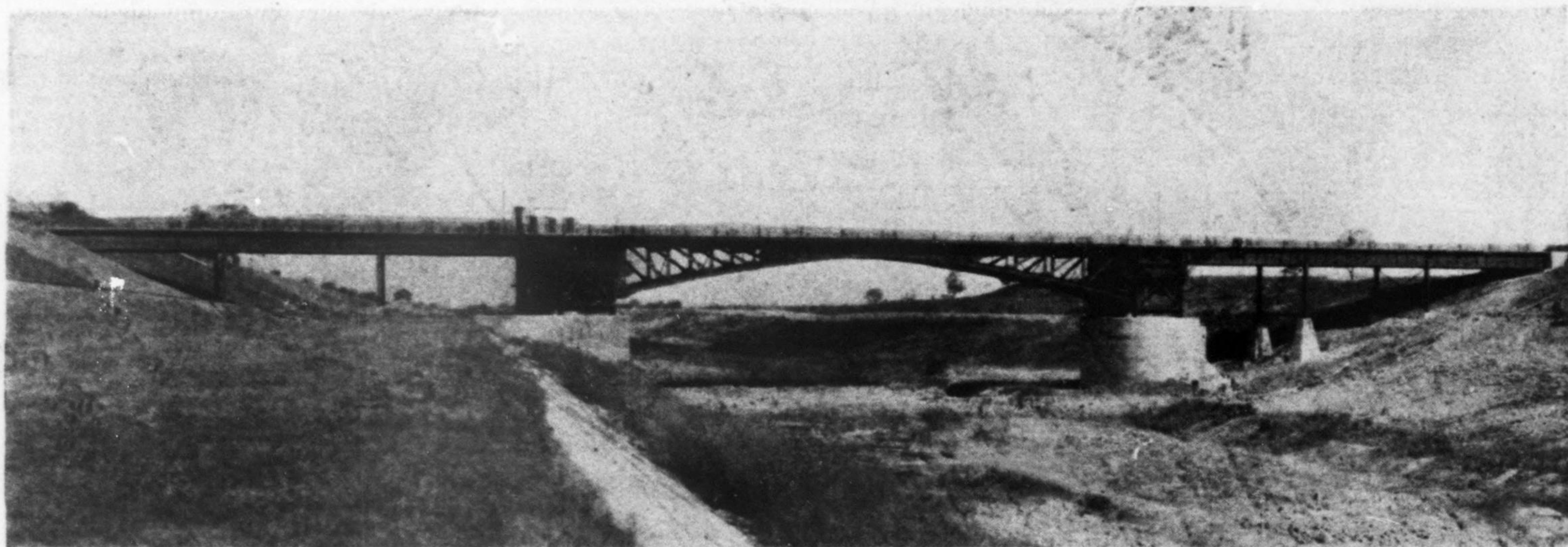
FIG. 12—BASCULE BRIDGE FOR THE HAMILTON-QUEENSTON HIGHWAY CROSSING
