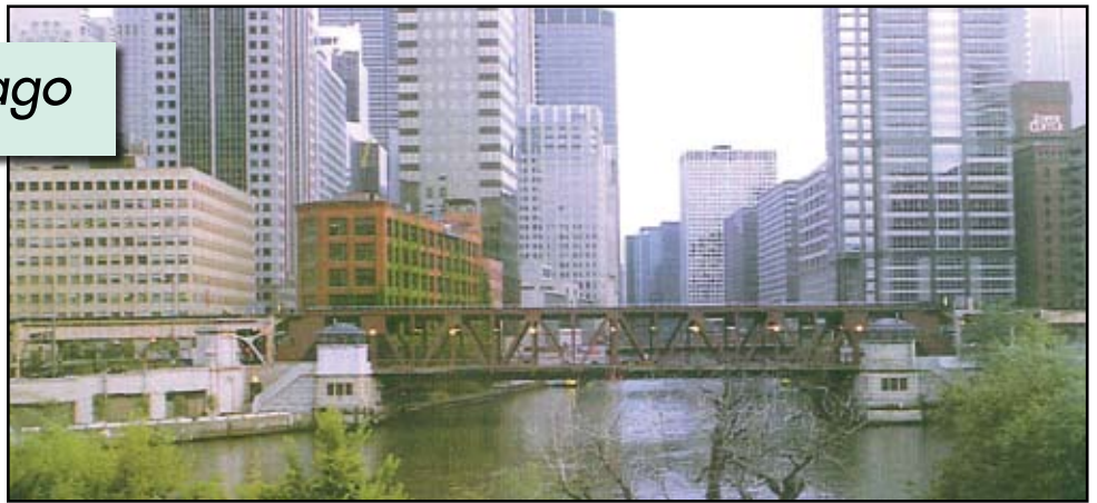
Lake Street Bridge, Chicago IL.
