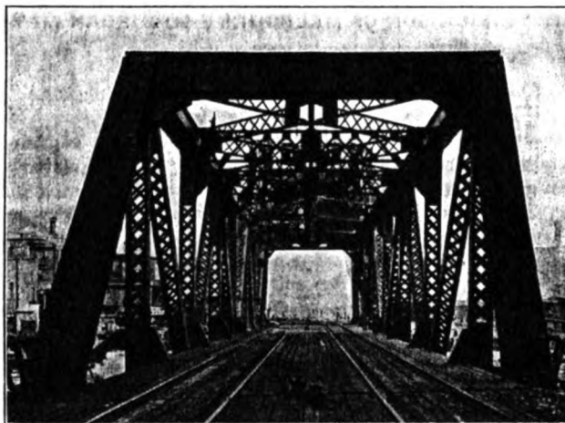
Portal View of Kinzie Street Bridge.
