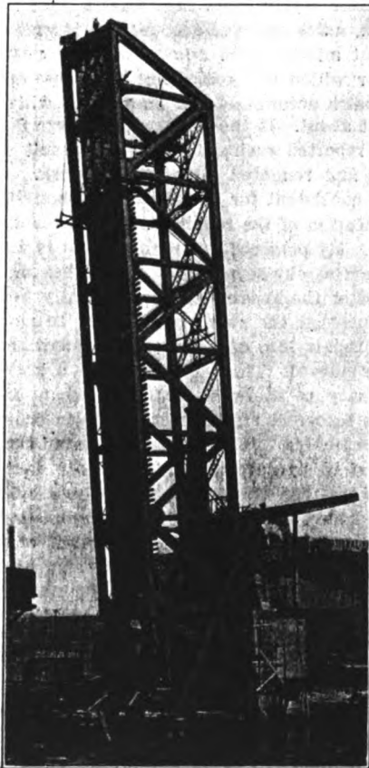
Side View of Kinzie Street Bridge.
