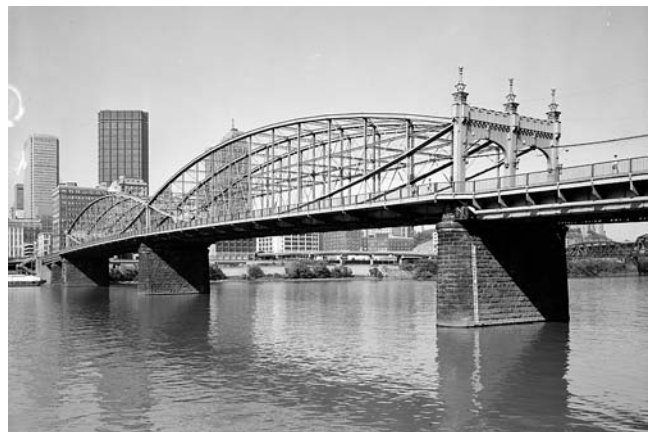
Figure 1. Smithfield Street, Pittsburgh, Pennsylvania. The trusses supporting the downstream lanes were completed in 1883. The upstream trusses date to 1891. Photo by Jack E. Boucher, 1974, HAER photograph PA-2-28.
