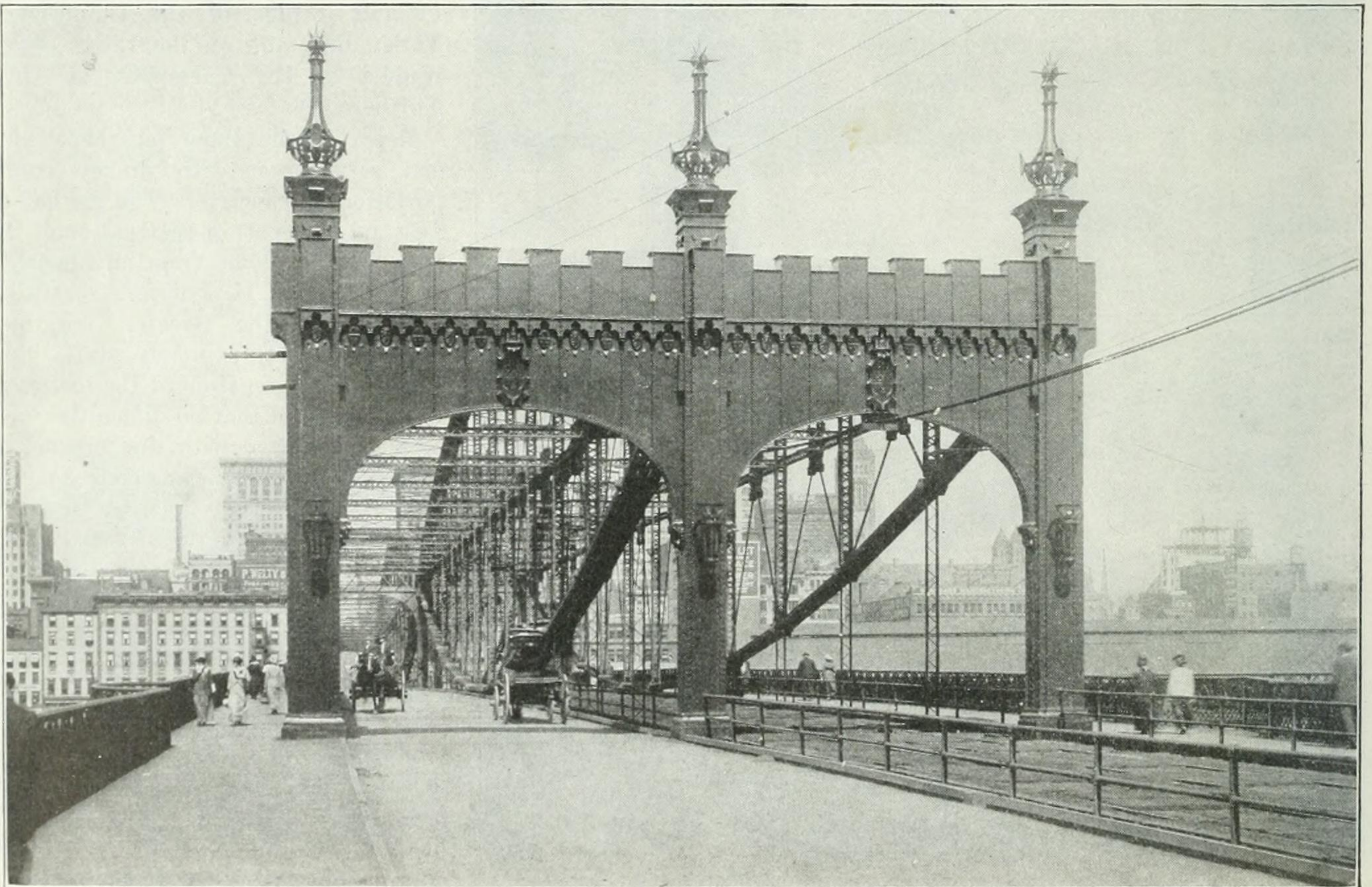
NEW SOUTH PORTAL OF SMITHFIELD ST. BRIDGE OVER MONONGAHELA RIVER, PITTSBURGH An ornamental structural-steel portal, replacing old cast-iron portals. The oldest part of the bridge dates from 1883
