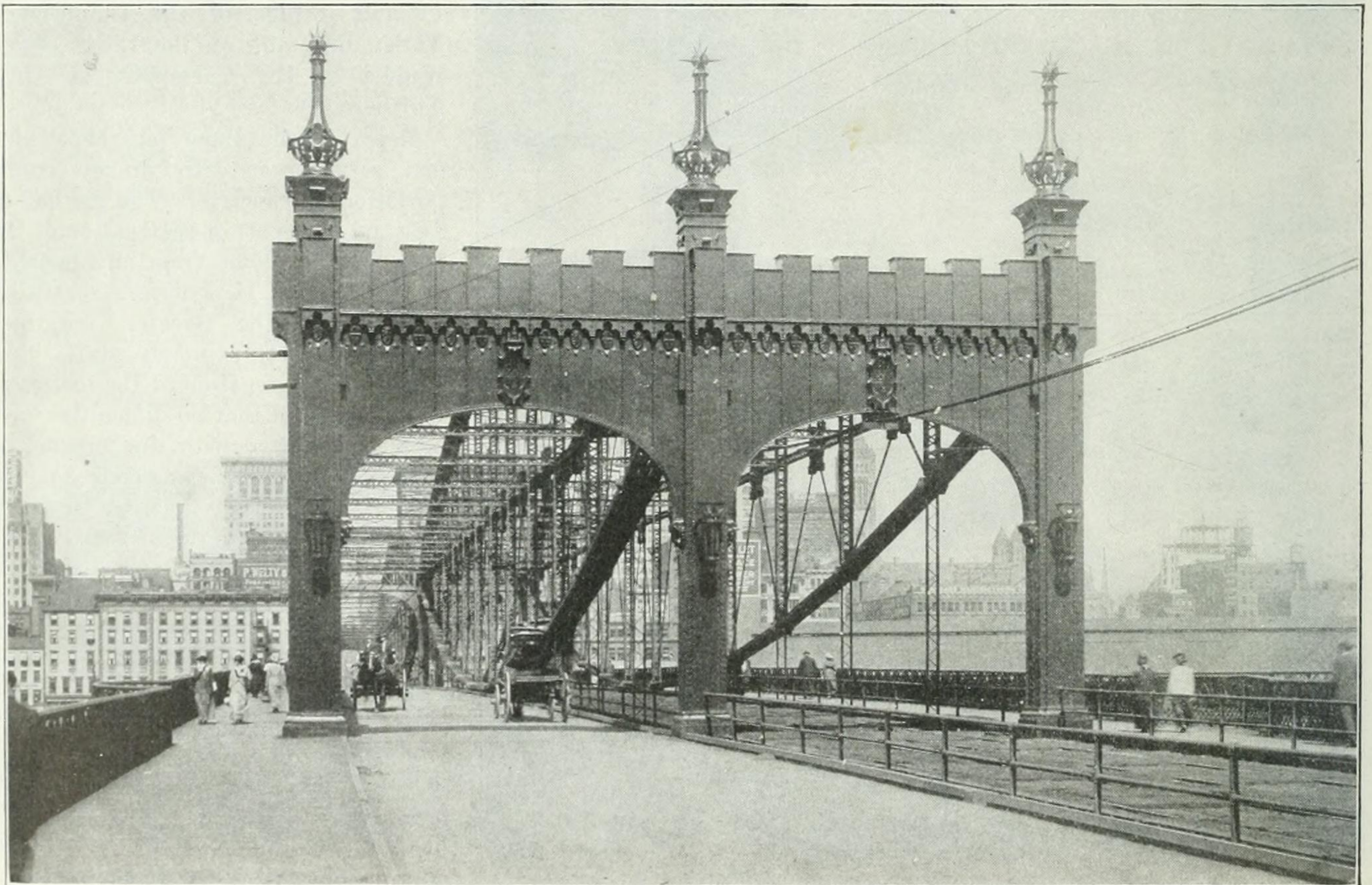
NEW SOUTH PORTAL OF SMITHFIELD ST. BRIDGE OVER MONONGAHELA RIVER, PITTSBURGH An ornamental structural-steel portal, replacing old cast-iron portals. The oldest part of the bridge dates from 1883
