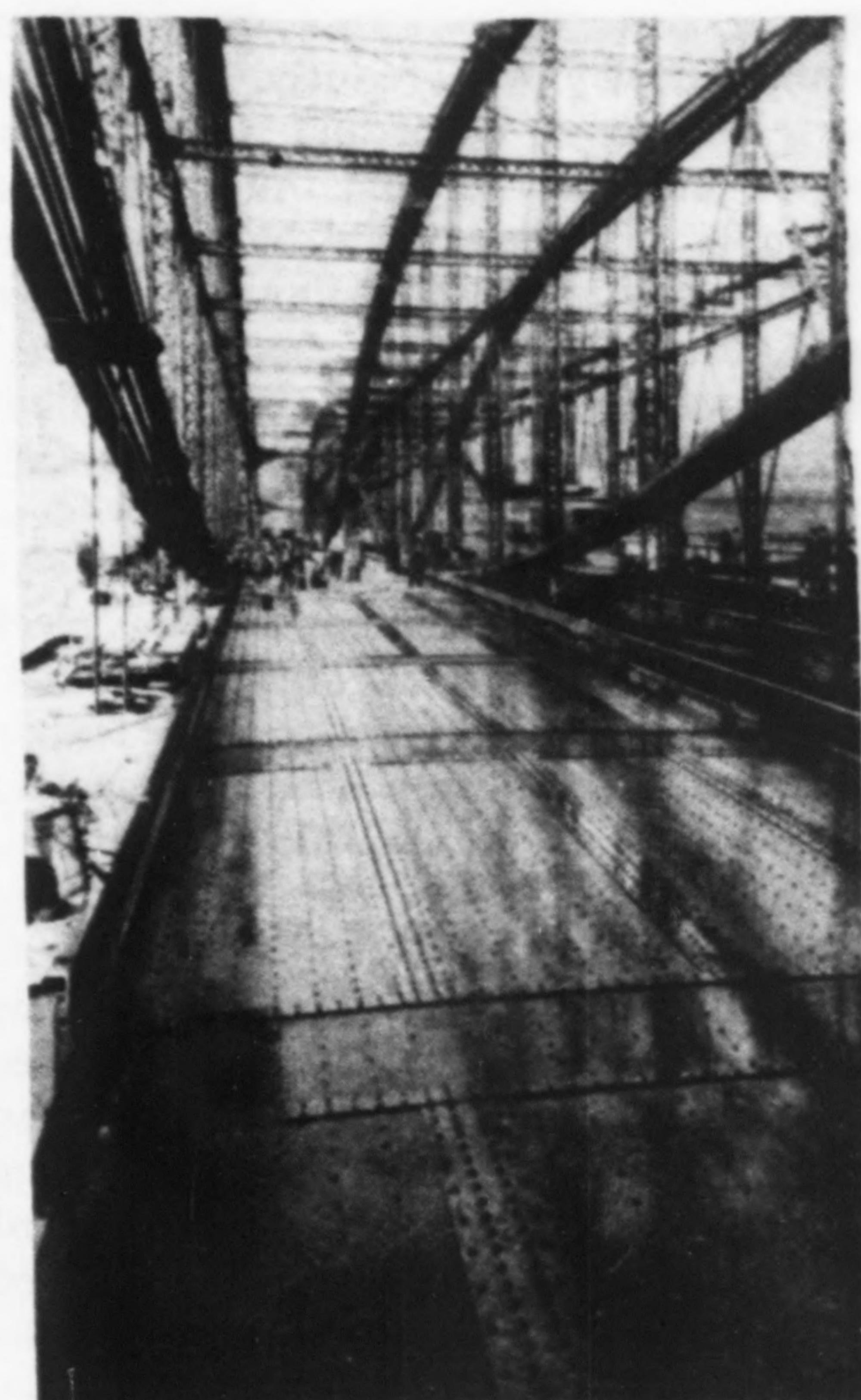
Fig. 4—The aluminum roadway floor ready for surfacing.
