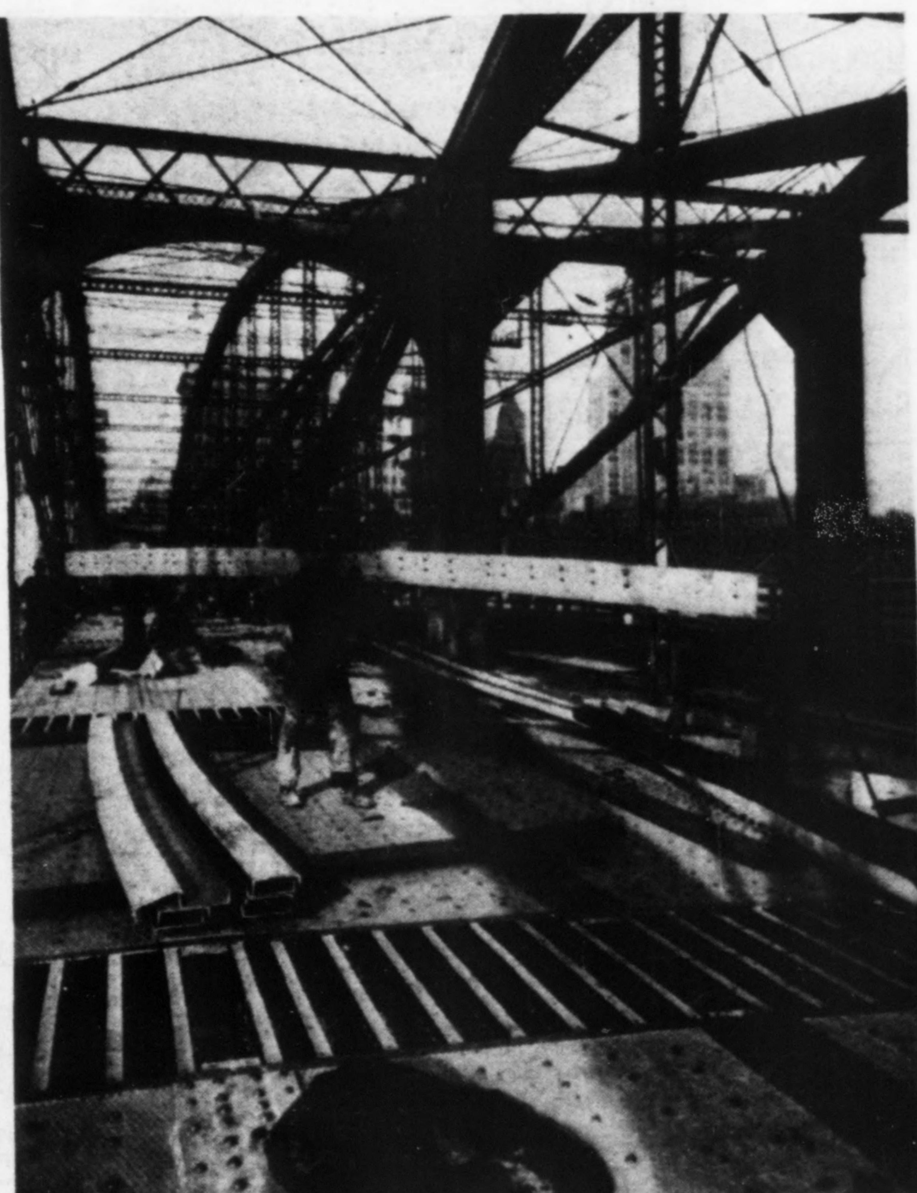
Fig. 1—By taking some 700 tons of dead weight from the load carried by its trusses, the old Smithfield St. Bridge in Pittsburgh, considered obsolete, was made capable of serving traffic for many years to come. The inherent lightness of aluminum and saving in deck weight through a novel ribbed slab of metal were prime factors in weight reduction.
