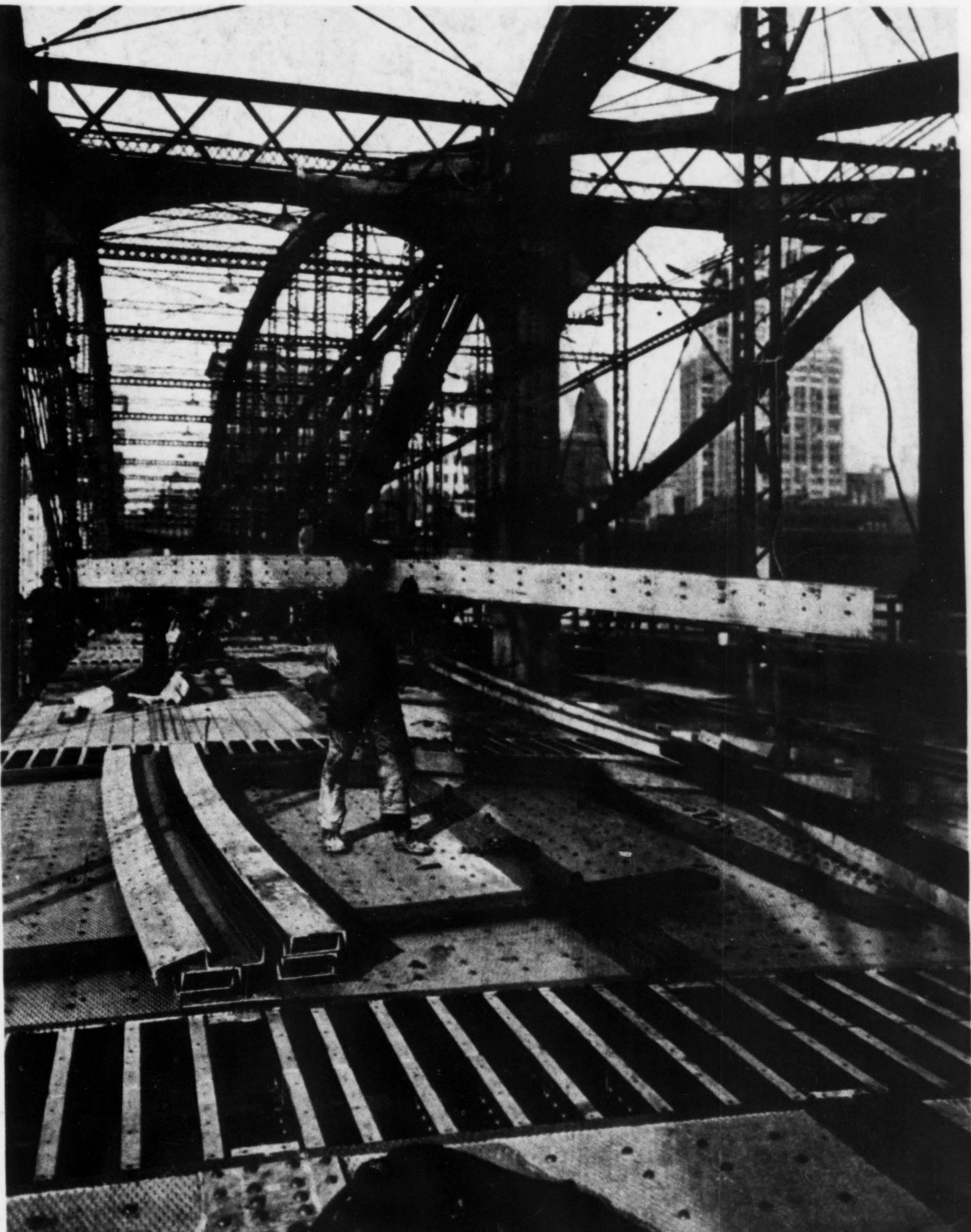
**THE FIRST APPLICATION OF ALUMINUM** to bridge construction has just been completed at Pittsburgh, Pa., where a new floor, including beams, stringers and deck, built entirely of aluminum alloy has been placed on the 51-year old Smithfield St. Bridge over the Monongahela River. A substantial dead load reduction permitted an increase in the safe live load, adding some 25 years to the useful life of the structure. Design and fabrication departed in no way from orthodox
