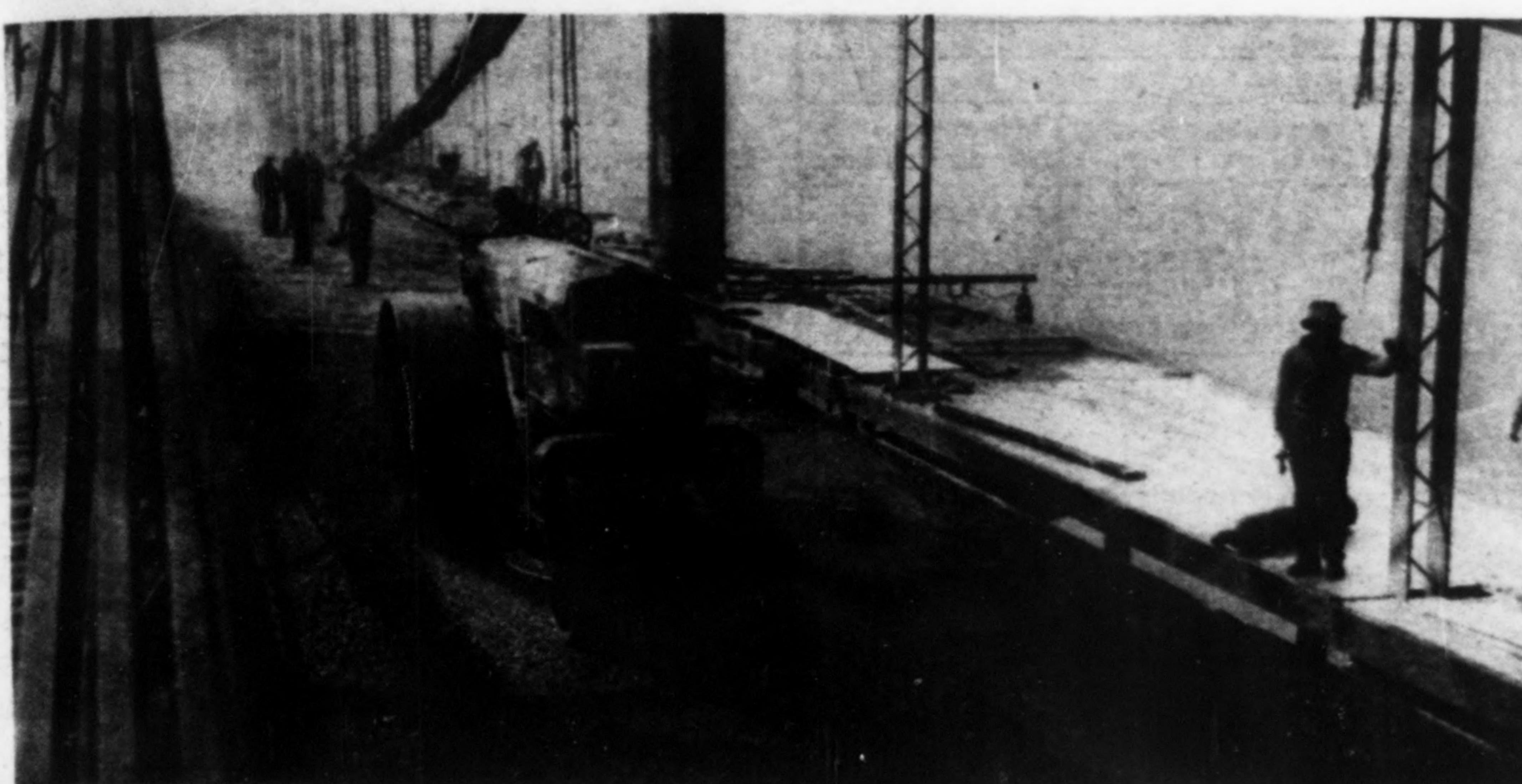
Fig. 8—Asphaltic surfacing laid on the roadway slab was compacted by rolling.
