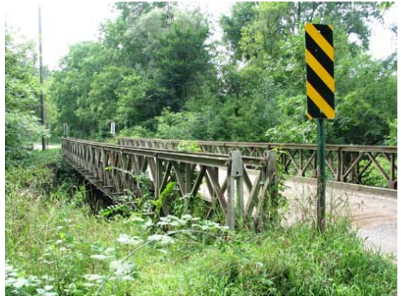
View of the Wilbur Road Bridge, facing west.
