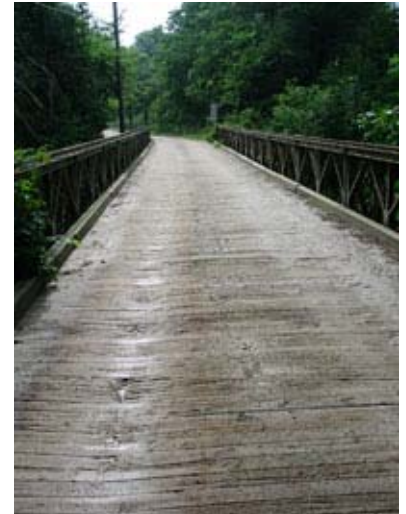
The wooden timber deck is showing telltale signs of 50+ years of wear.
