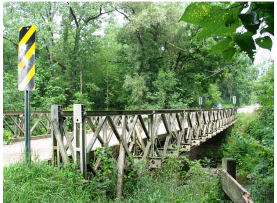
View of the steel trusses, facing east.
