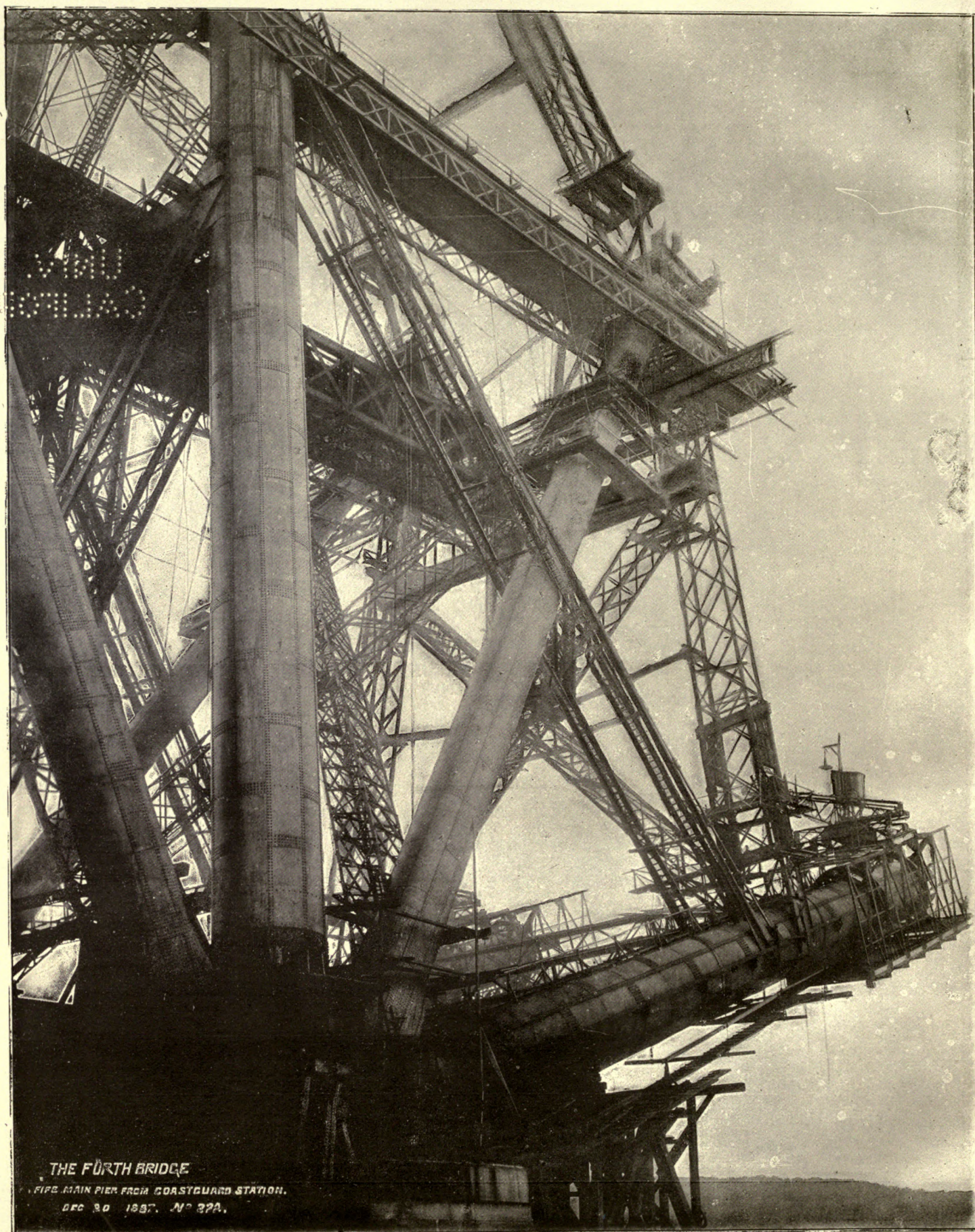
FIVE PIER. LOWER HALF OF FIRST BAY IN FIXED CANTILEVER.
