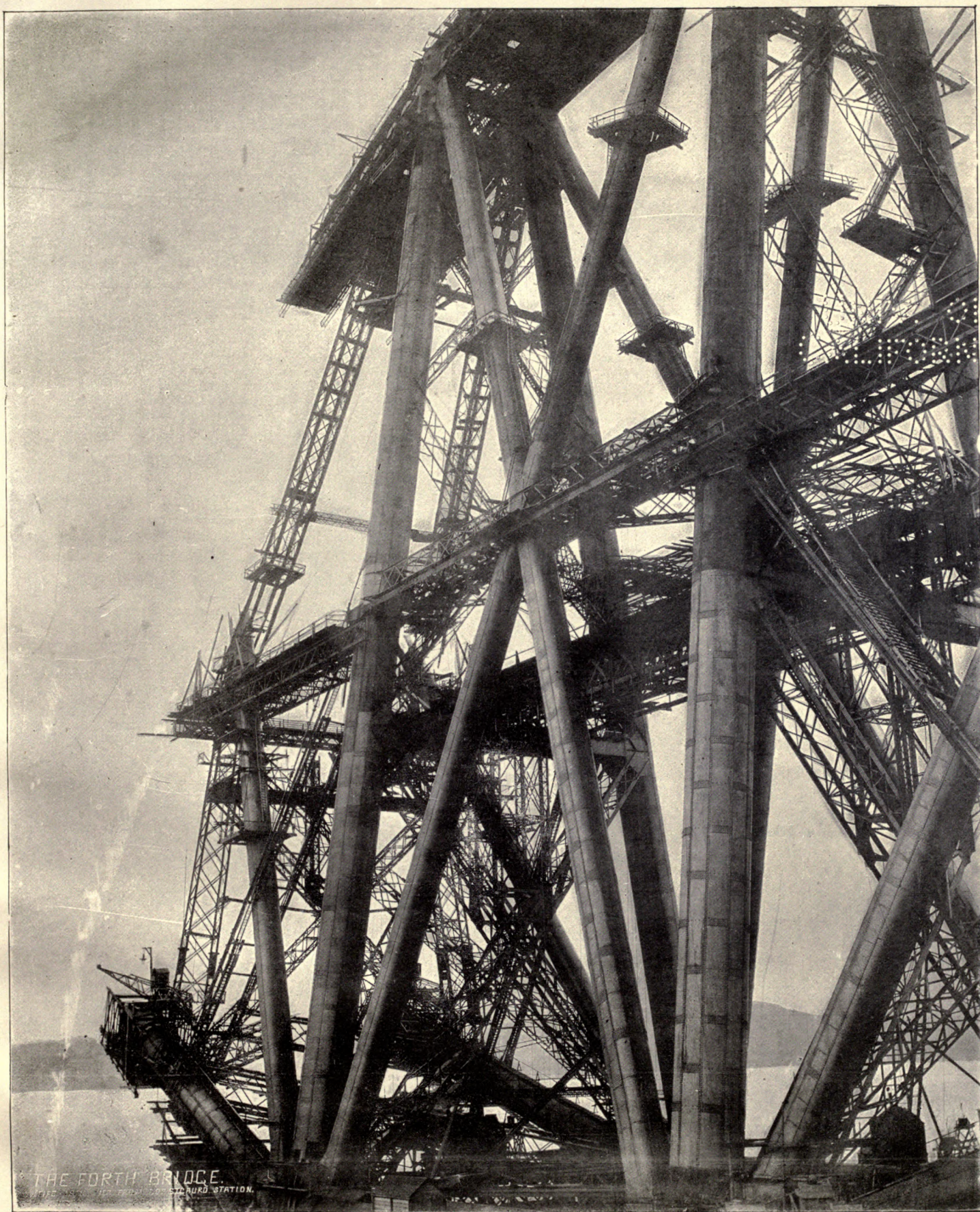
FIVE PIER. CENTRAL TOWER AND LOWER HALF OF FIRST BAY IN FREE CANTILEVER.
