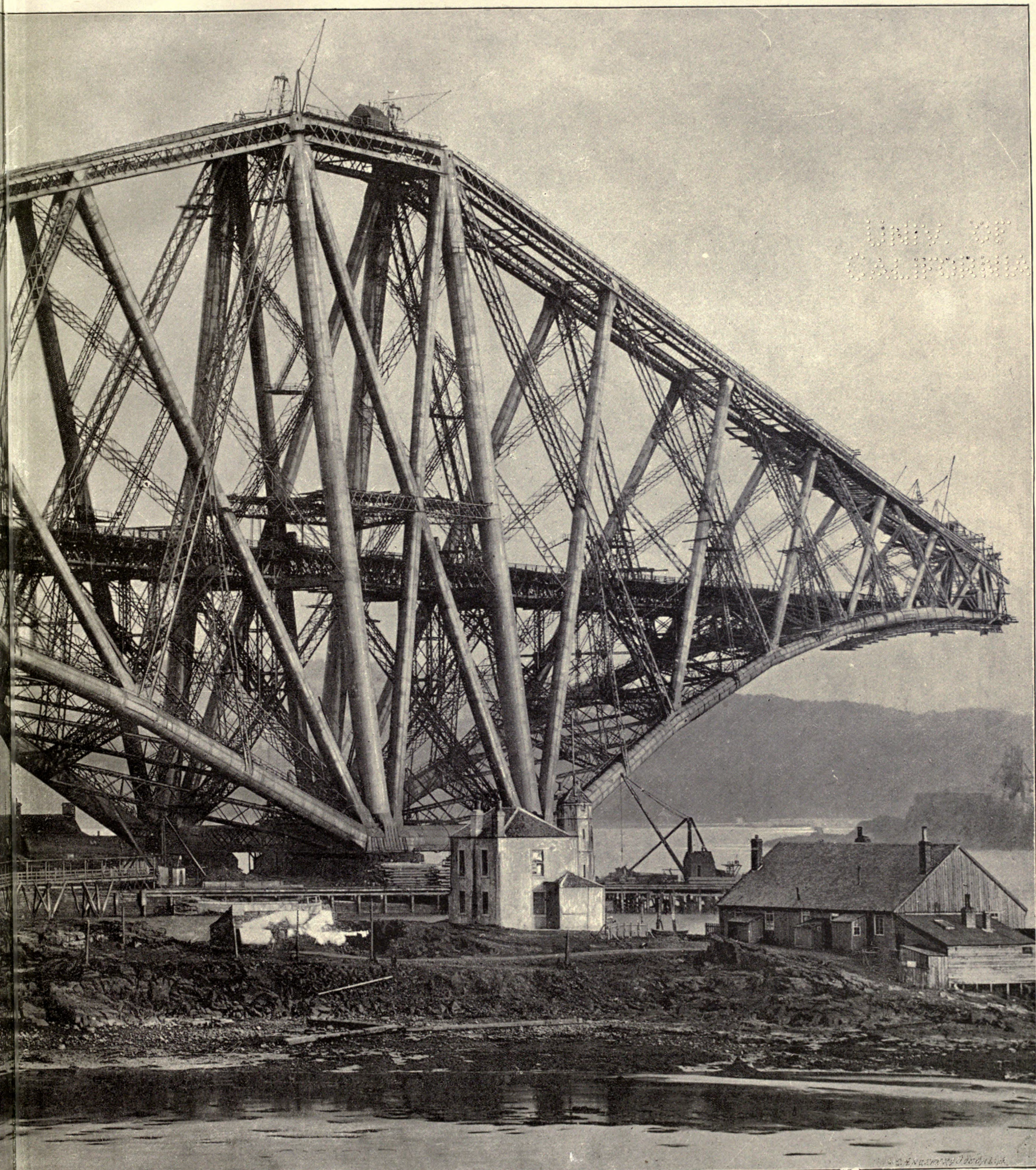
CONSTRUCTION COMMENCED ; FIXED CANTILEVER NOT QUITE COMPLETED.
