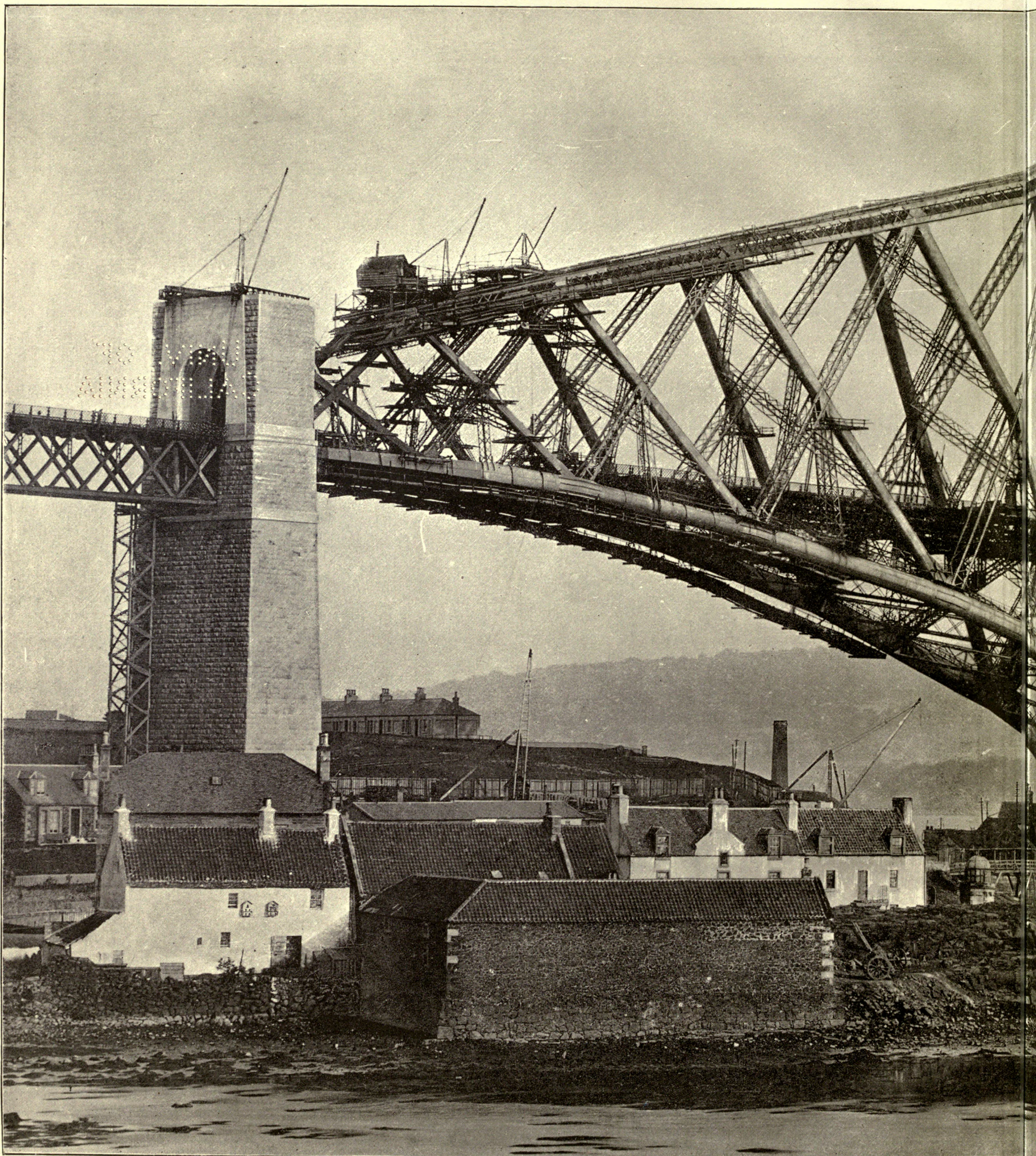
FIFE PIER. FREE CANTILEVER COMPLETED AND CENTRAL GIRDER
