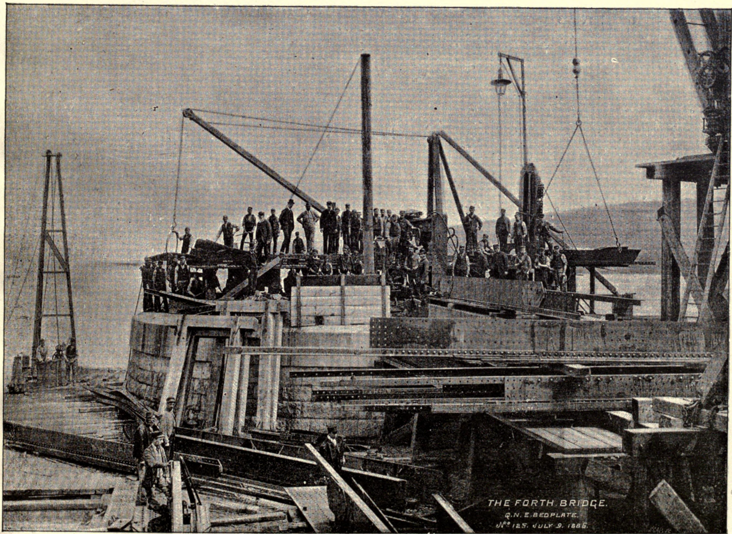
QUEENSFERRY NORTH-EAST PIER. PUTTING TOGETHER UPPER BEDPLATE.
