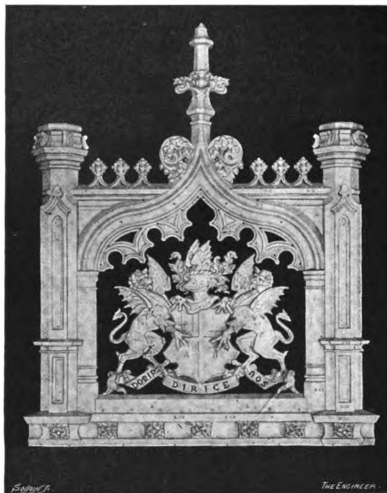
Fig. 62—CITY ARMS, HIGH-LEVEL FOOTWAY
