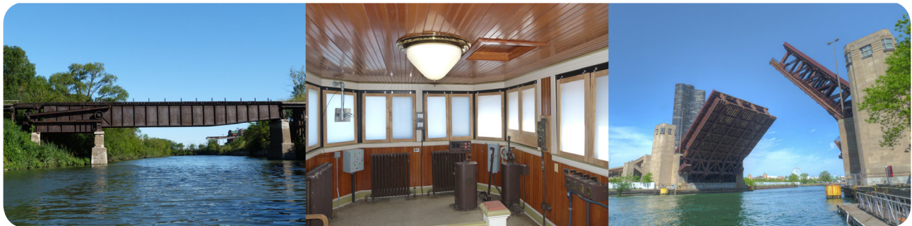
Above from left to right: Chicago and Illinois Western Railway Rall Bascule Bridge, Lake Street Bridge bridgetender house, and Lake Shore Drive Bridge. Photos by Nathan Holth.
