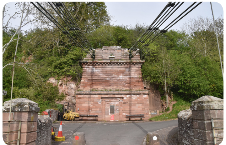
The east end of the bridge has no free-standing tower. Instead, a stone structure built into a natural cliffside serves as both tower and anchorage. The road turns to the right here. Photo by Nathan Holth.
