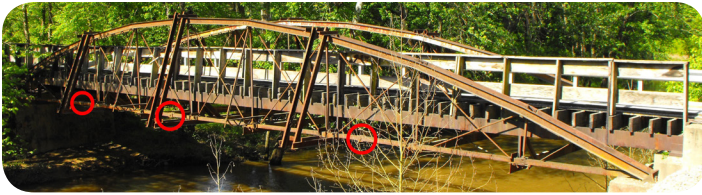
Above: Red circles show where the pins on the lower chord occur. Below: Lower chord pin connection detail. Photos by Nathan Holth.
