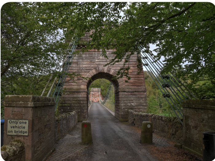
View looking east showing the arched tower and the small anchorages in front. Photo by Nathan Holth.
