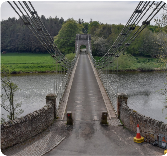
A view looking west at the bridge, taken from the lower ledge of the east anchorage. Photo by Nathan Holth.
