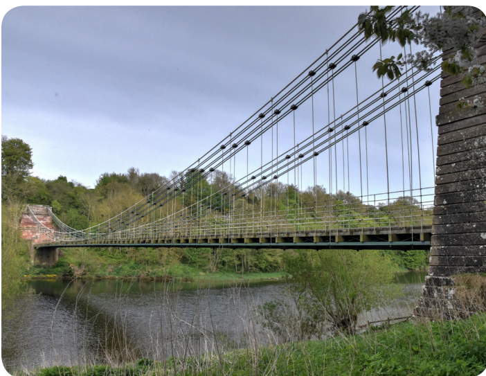
View beside the bridge facing southeast toward England. Photo by Nathan Holth.
