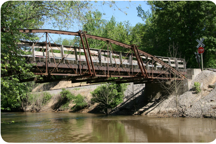
Bridge #150. Photo by Nathan Holth.
