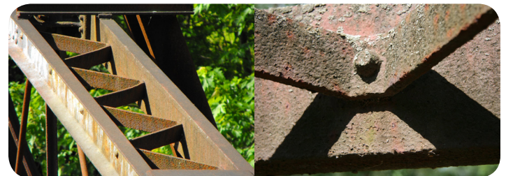
Detail showing the "continuous trussing" in the chord. Photo by Nathan Holth.
