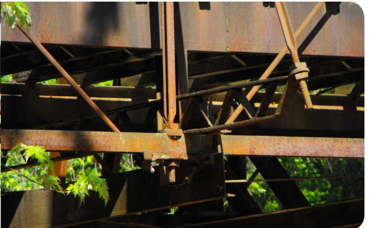
Perpendicular brace beams that extend beyond the trusses and anchor the sway braces. Photo by Nathan Holth.
