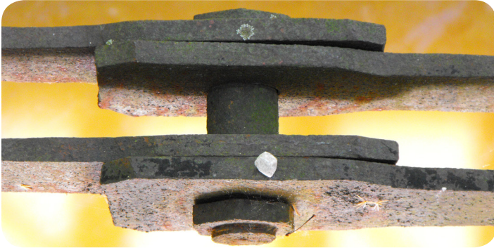
Above: Red circles show where the pins on the lower chord occur. Below: Lower chord pin connection detail. Photos by Nathan Holth.
