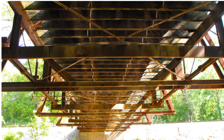
Perpendicular brace beams that extend beyond the trusses and anchor the sway braces. Photo by Nathan Holth.
