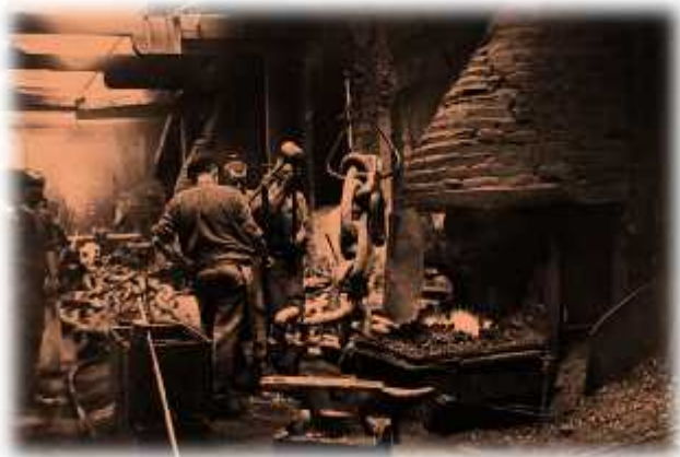
Chainsmiths at work at Newbridge
