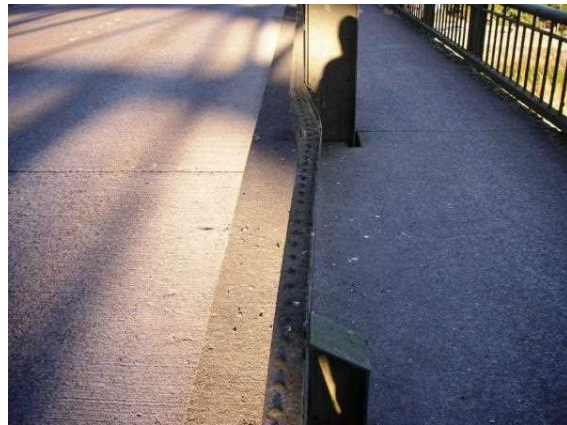
Traffic barrier rail, sidewalk, and outer handrail.
