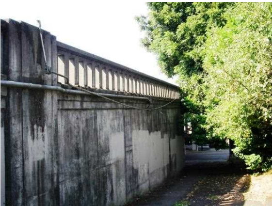
Curtain wall & rail on east approach.
