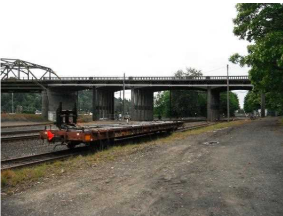
East approach over railroad tracks N.
