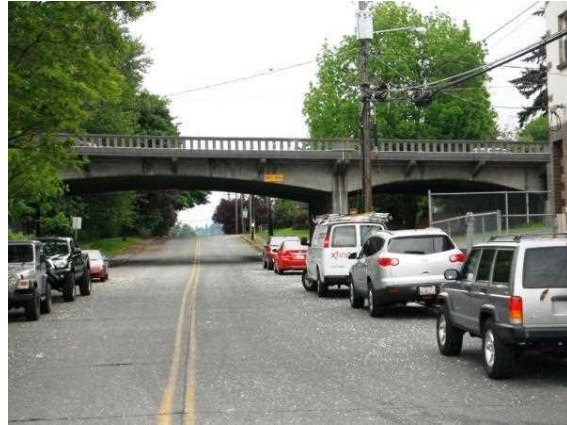
East approach over First Ave.
