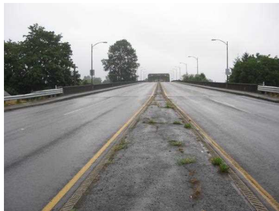
West approach deck to E.
