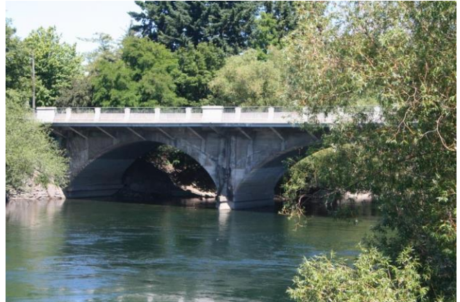
View to the northwest Bridge, south side 2013
