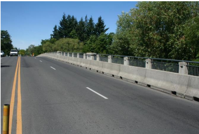
View to the northwest Bridge deck and north balustrade 2013
