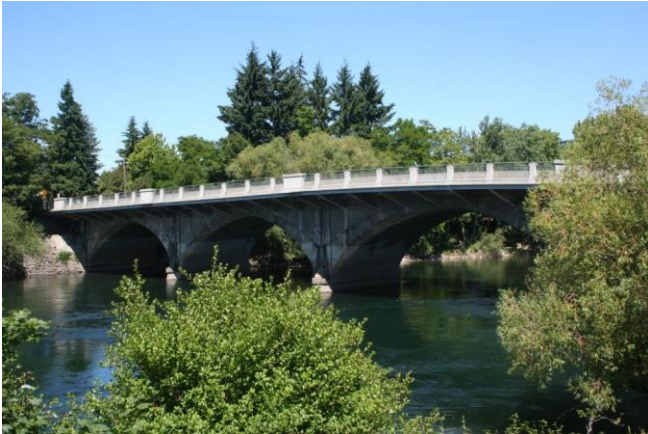
View to the northwest Bridge, south side 2013
