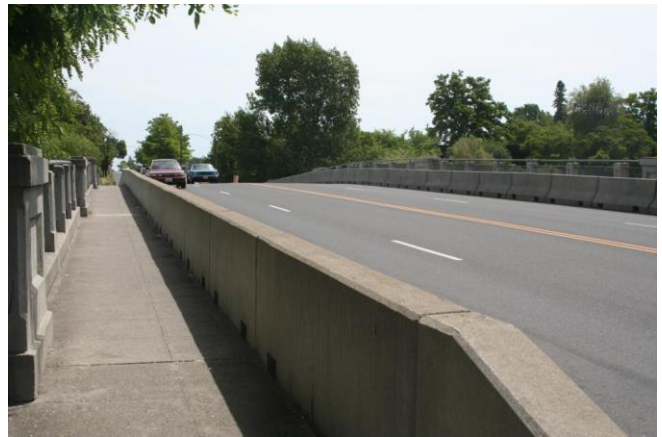
View to the southeast Bridge deck, west approach 2013
