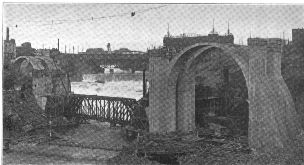
Erecting Falsework for Monroe Street Arch Bridge; Steel Trusses in Place.
