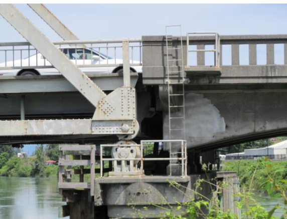
Swing unit seat on pier joining east approach
