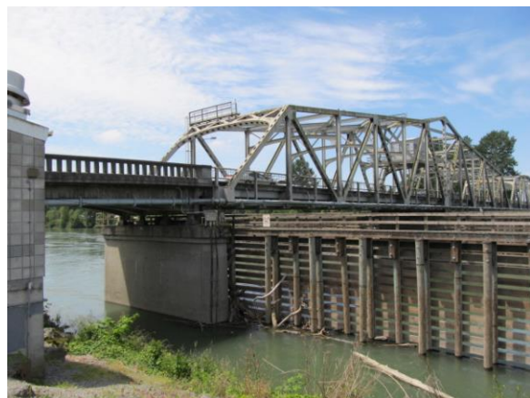
East pier and timber fender
