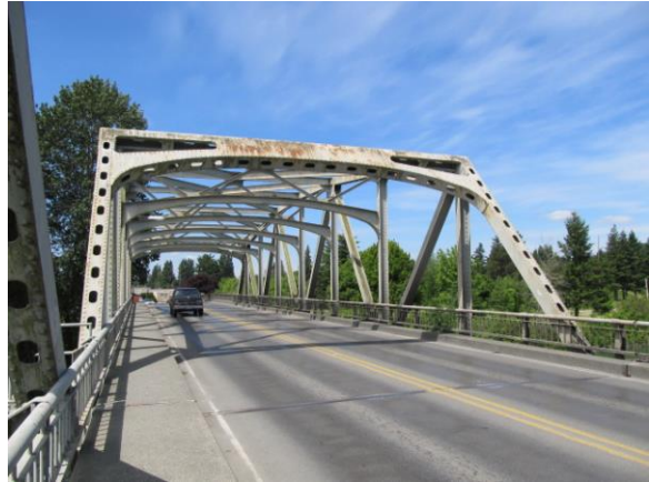
East portal of fixed Warren span 2011
