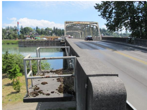
Cantilevered platform N side W approach 2011
