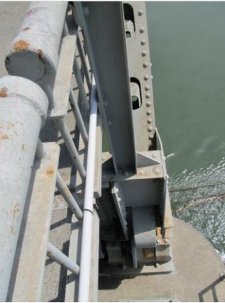
Swing unit seat south side west end 2011
