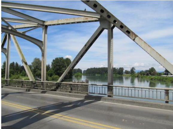
East portal vertical column & railing 2011
