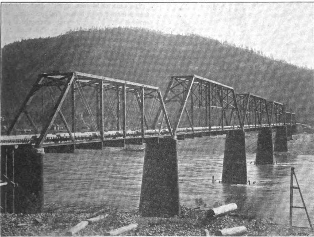
COMBINATION BRIDGE AT NORTHPORT.
