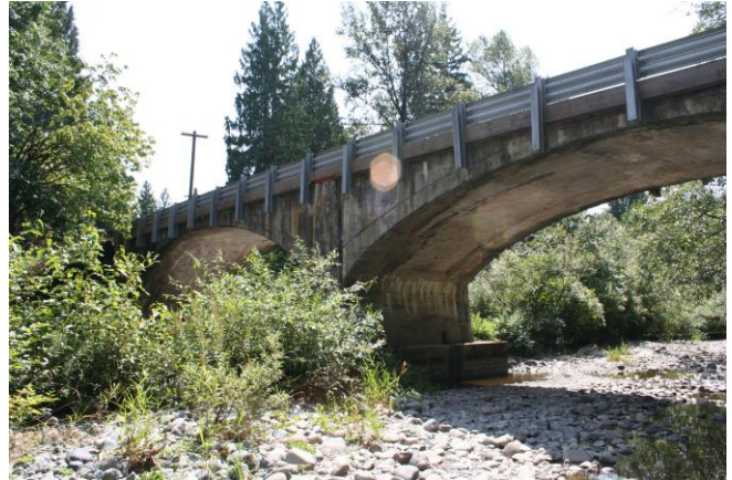
View to the south Northeast side of bridge
