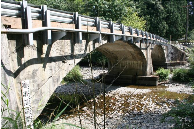
View to the east Southwest side of bridge
