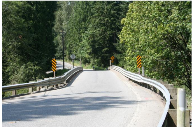
View to the northwest Southeast approach
