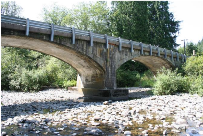
View to the west Northeast side of bridge
