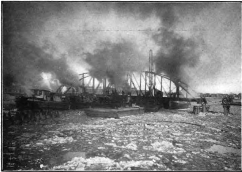
Fig. 5.—The Bridge Being Landed.
