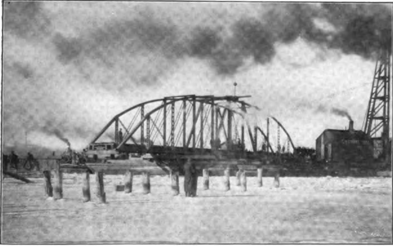
Fig. 4.—The Bridge Starting.
