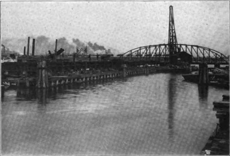
Fig. 17.—Bridge Floor During Erection.
