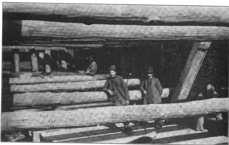
Fig. 8.—Abutment Cofferdam.
