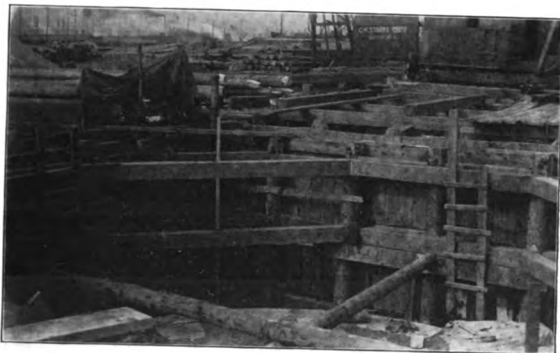
Fig. 7.—Center Pier Cofferdam.
