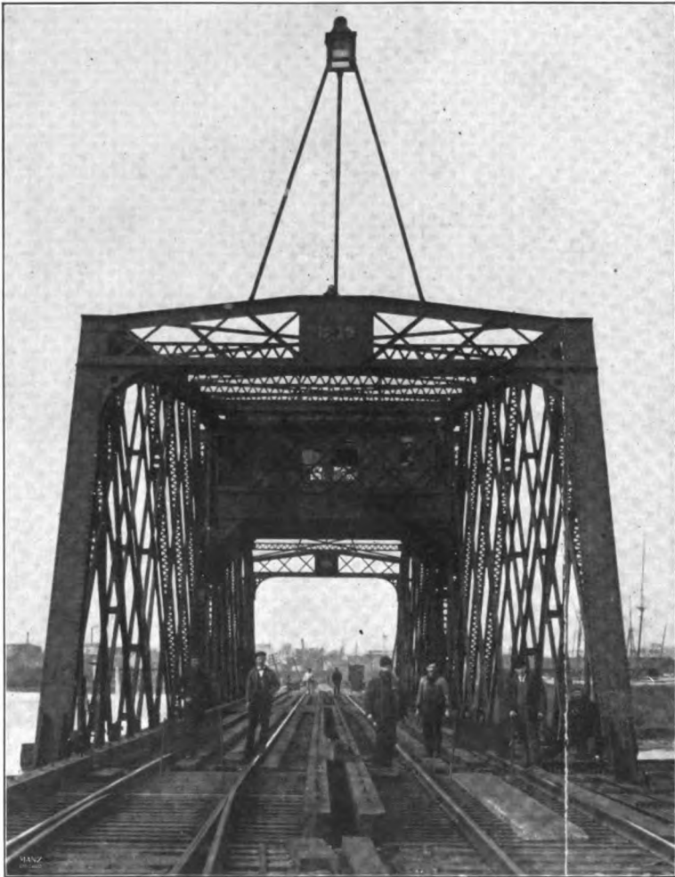
Fig. 12.—End View of Bridge.
