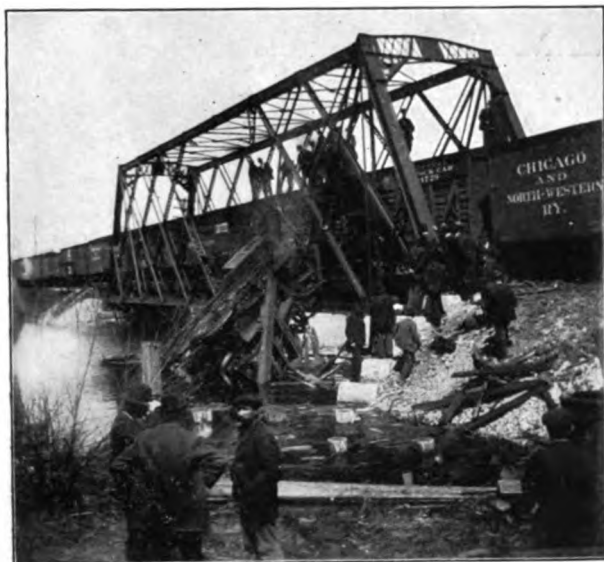
Fig. 13.—Accident to Bridge at Fond du Lac.
