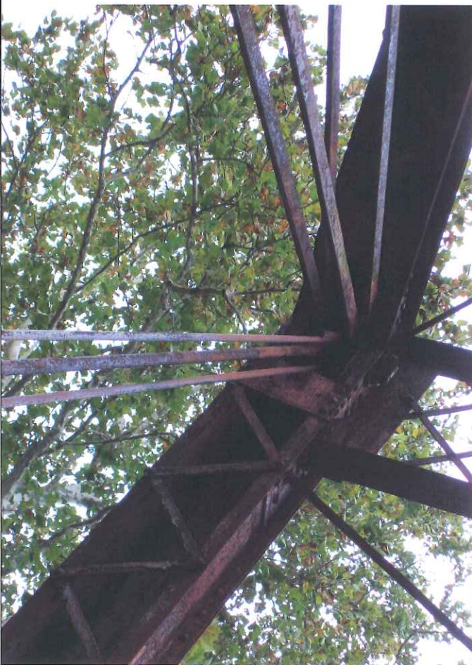
10. View of endpost connection.
