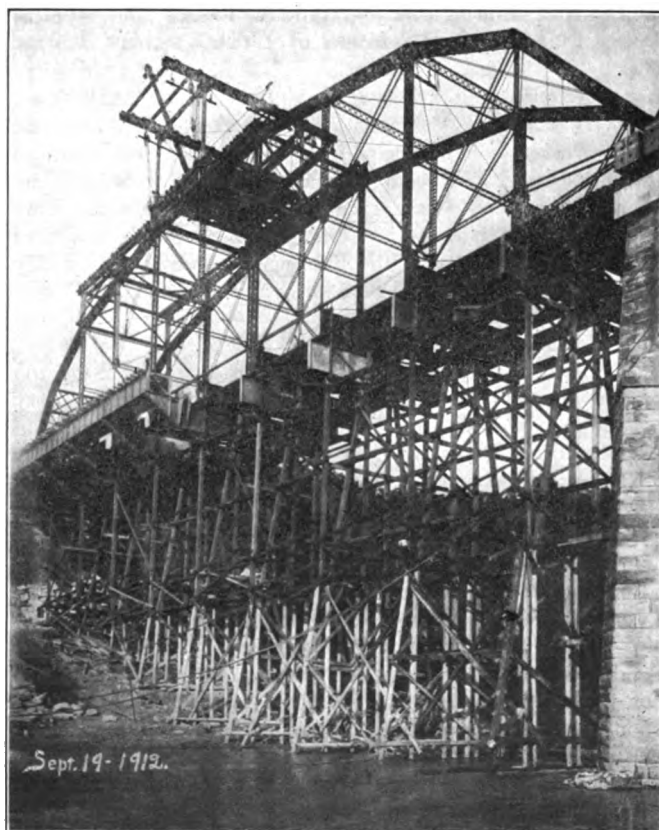
Fig. 12—False Work Under Span 5 Showing Connection of New Floor Beams to Old Ones and the Brackets Supporting Material Track.
