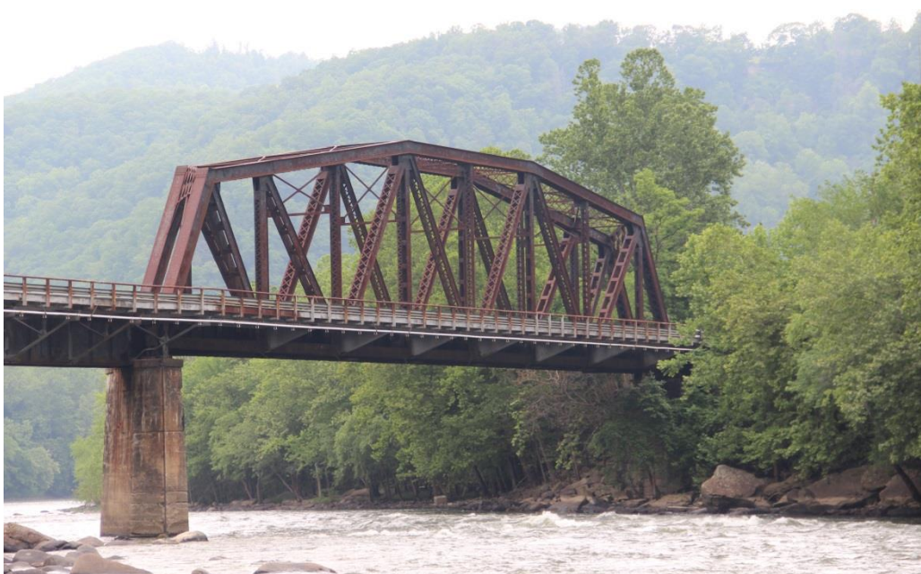
Photo 22: East profile of main Warren truss span, facing northwest.
